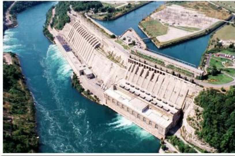
Figure 1.3: Niagara Fall Hydro Power Plant
