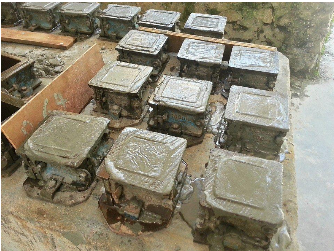
Figure 3.10: Casting of Concrete
