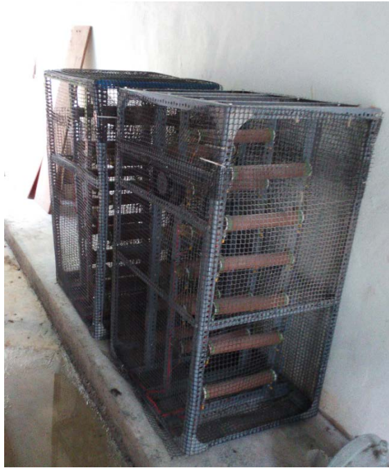
Figure 3.3 Load emulator installed at the laboratory
