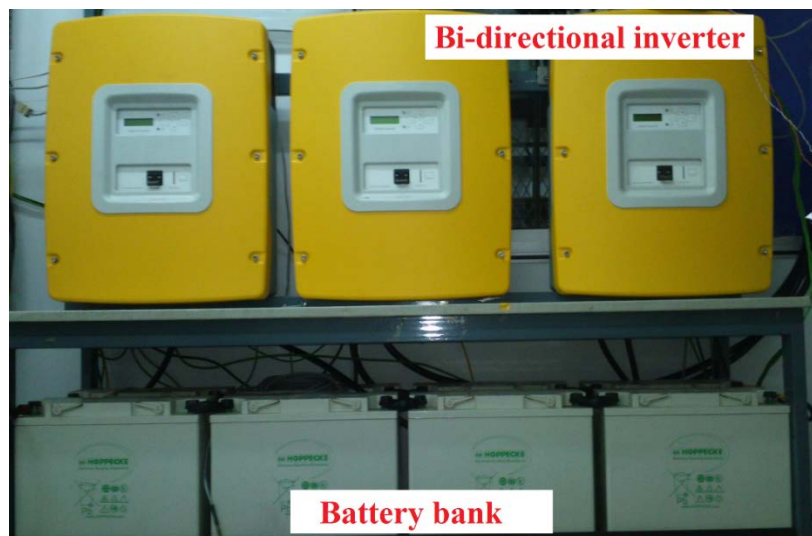
Figure 3.5 Three units of bi-directional inverter integrated with batteries
