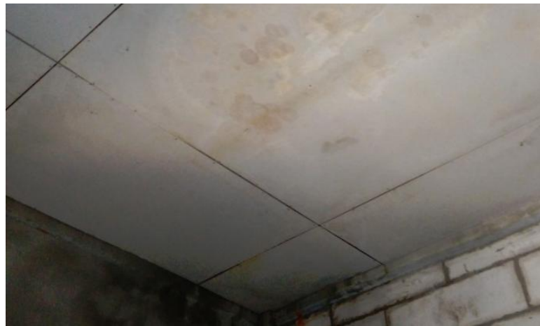
Figure 4.5: Concrete ceiling of the Experimental Residential Room
