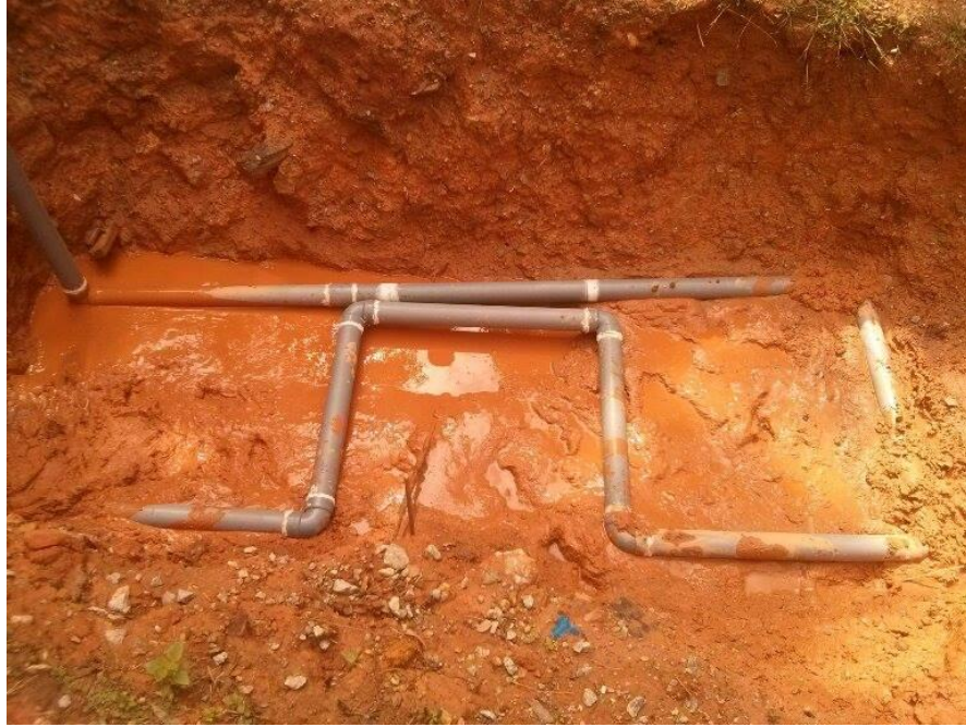
Figure 4.34: Actual EAHE Pipe Layout on Site
