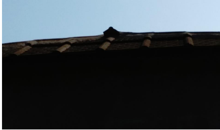
Figure 4.4: Roof tiles of the Experimental Residential Room
