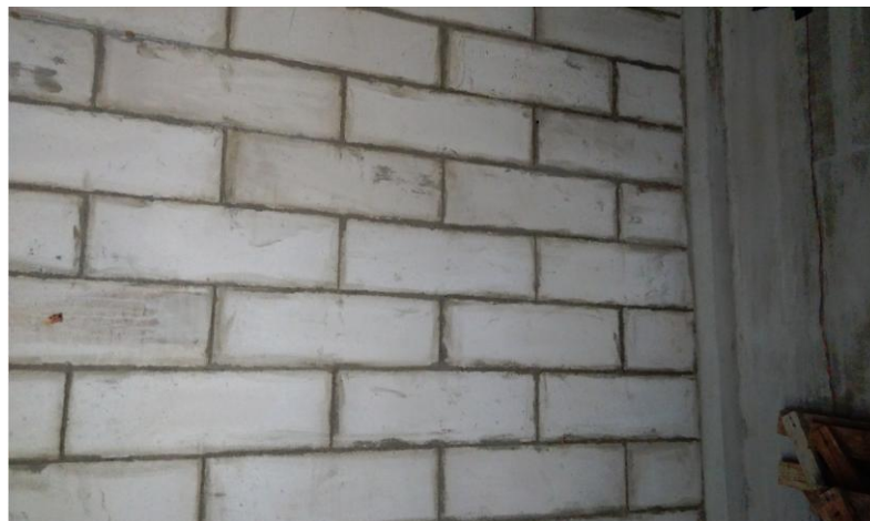
Figure 4.6: Walls of the Experimental Residential Room
