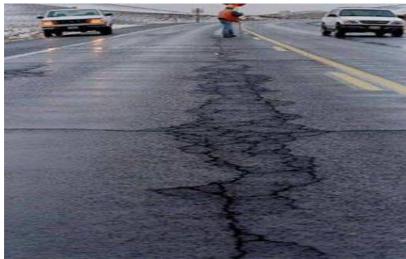
Figure 1.1: Fatigue cracking (theconstructor.org, 2011)
