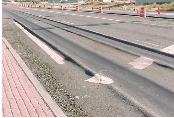
Figure 1.2: Rutting (Pavement interactive, 2008)
