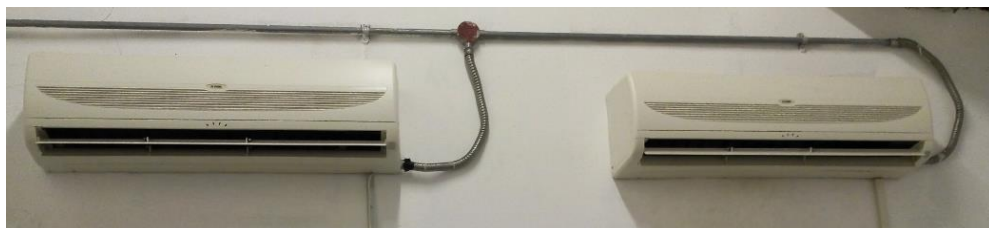
Figure 4.45: Indoor air exchange unit
