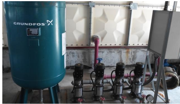
Figure 4.57: Water pump
