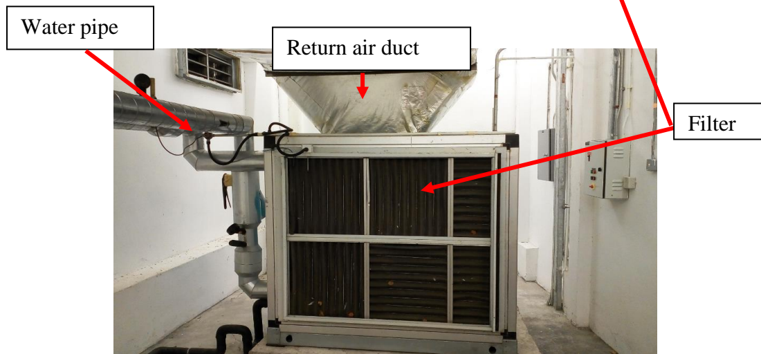
Figure 4.28: AHU filter
