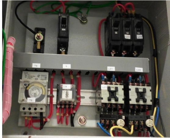
Figure 4.48: Switch box timer control
