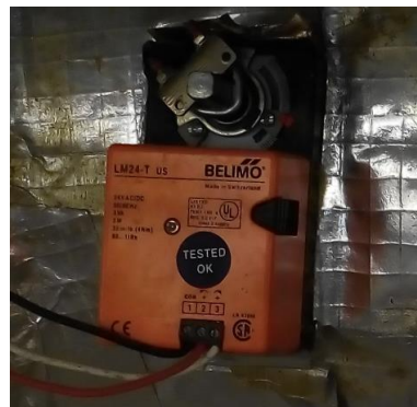
Figure 4.38: HVAC electric air flow on off control
