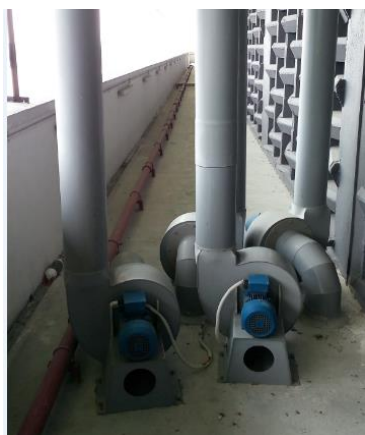
Figure 4.54: Fume exhaust fan
