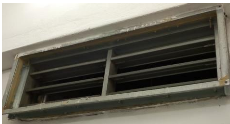
Figure 4.43: Return vent grille
