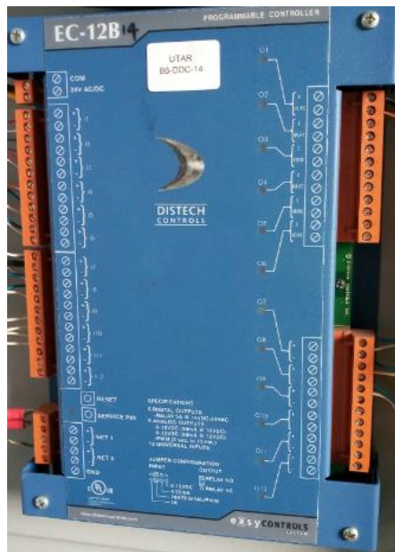
Figure 4.49: DISTECH Control module/VSD
