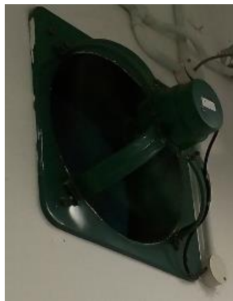
Figure 4.55: Indoor exhaust fan
