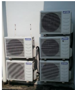
Figure 4.46: Outdoor condenser unit
