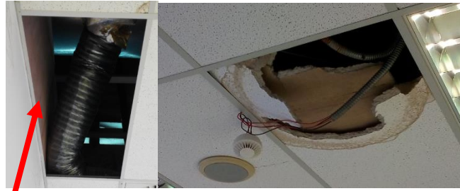
Figure 4.61: uncover ceiling / spoiled ceiling
