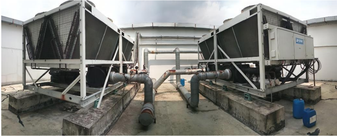
Figure 4.34: HVAC condenser units
