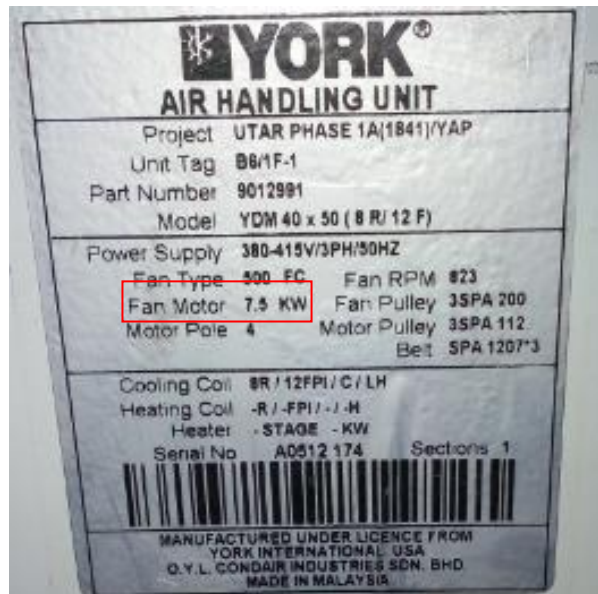
Figure 4.31: AHU information lable
