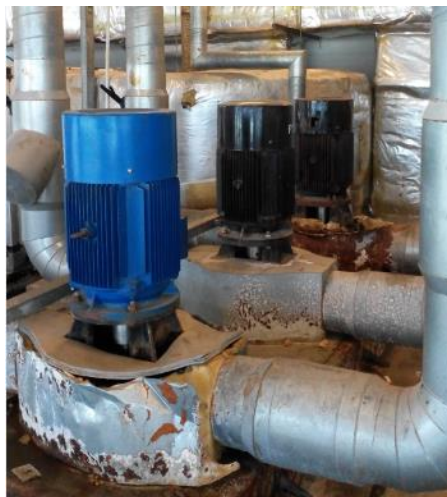
Figure 4.32: Water pump for HVAC
