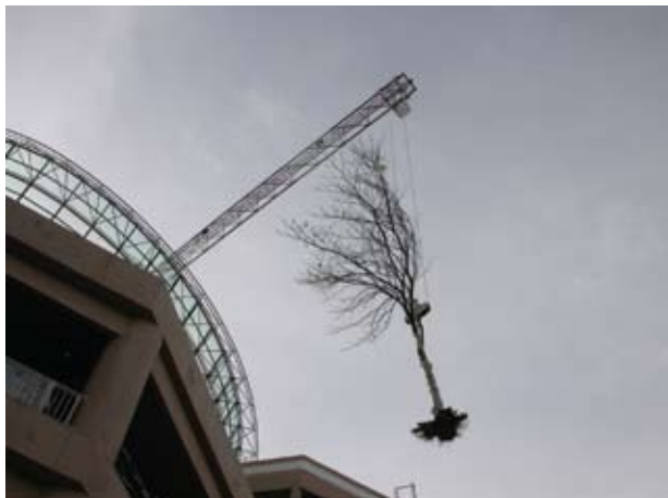
Lifting the tree above the roof
