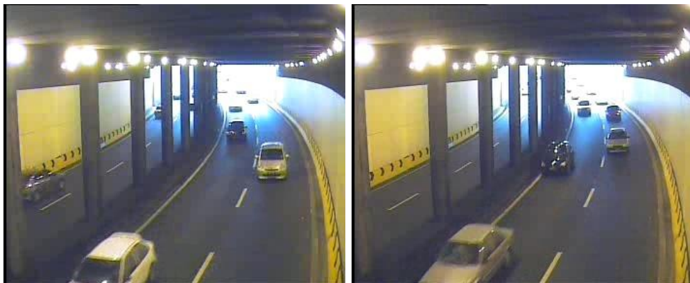
Video 2: Inside the tunnel, where the entrance is covered in high brightness
