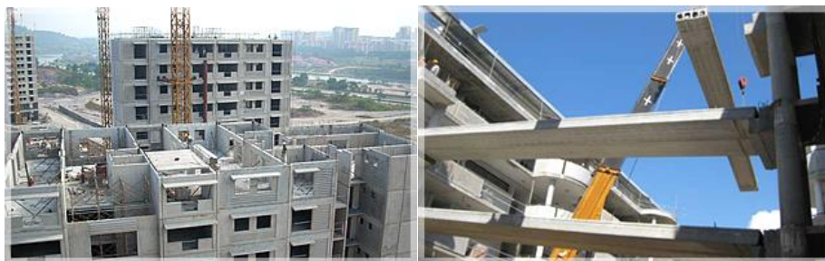
Figure 2.1: Precast Concrete System (source: Eastern Pretech (Malaysia) Sdn Bhd)
