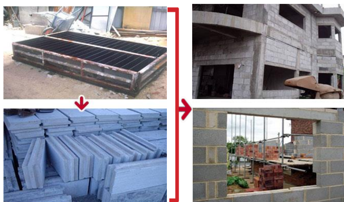
Figure 2.5: Blockwork System (source: Fast Build Sustain Sdn. Bhd.)
