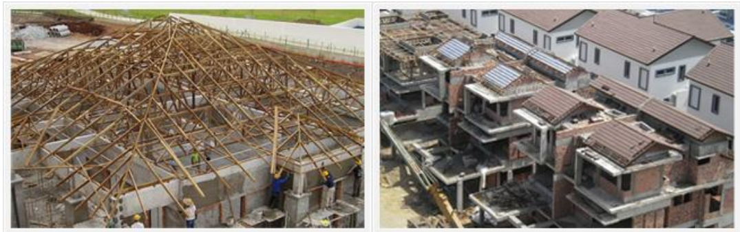
Figure 2.4: Prefabricated Timber Roof at Setia Pearl Island (source: Setia - Wood Industries Sdn Bhd)
