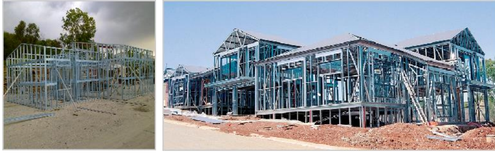
Figure 2.3: Steel Framing System (source: Superdaya Group)
