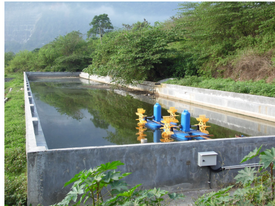
Leachate treatment pond
