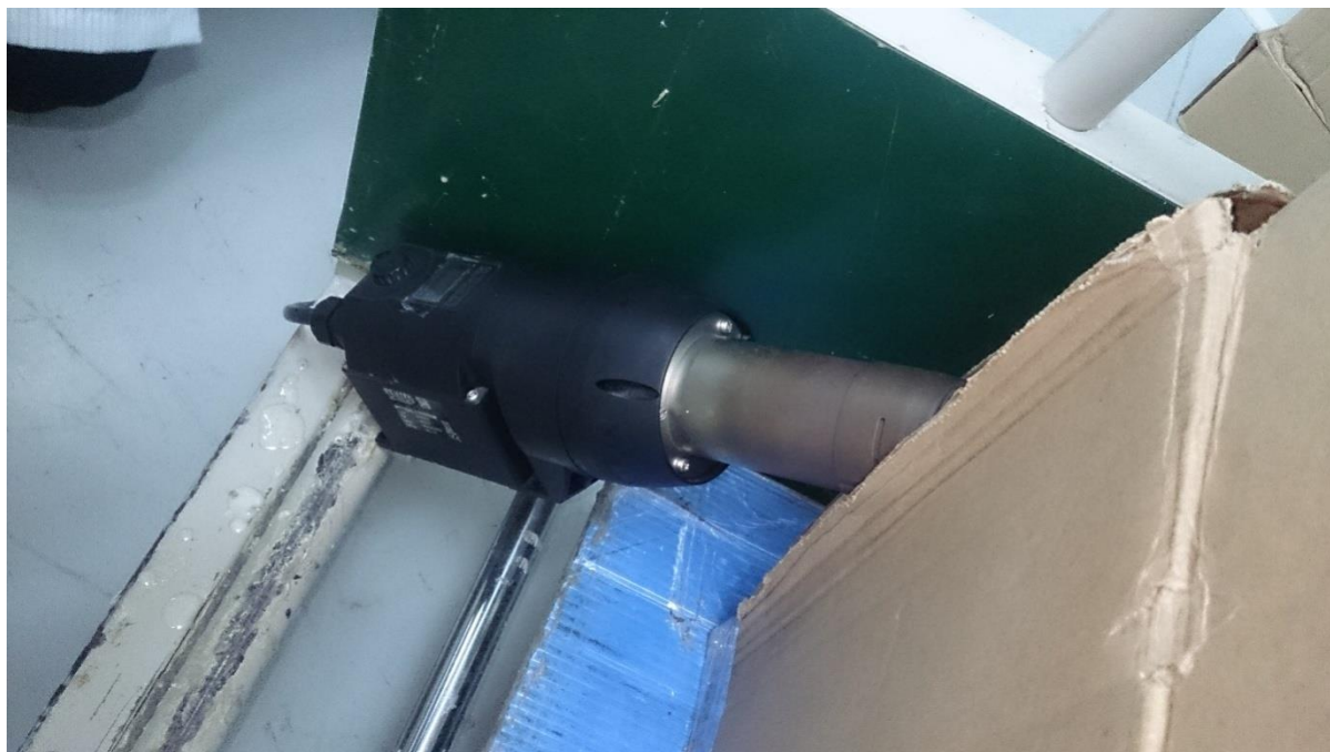
Figure 4.36: Hot Air Blower Used to Speed Up the Curing Process
