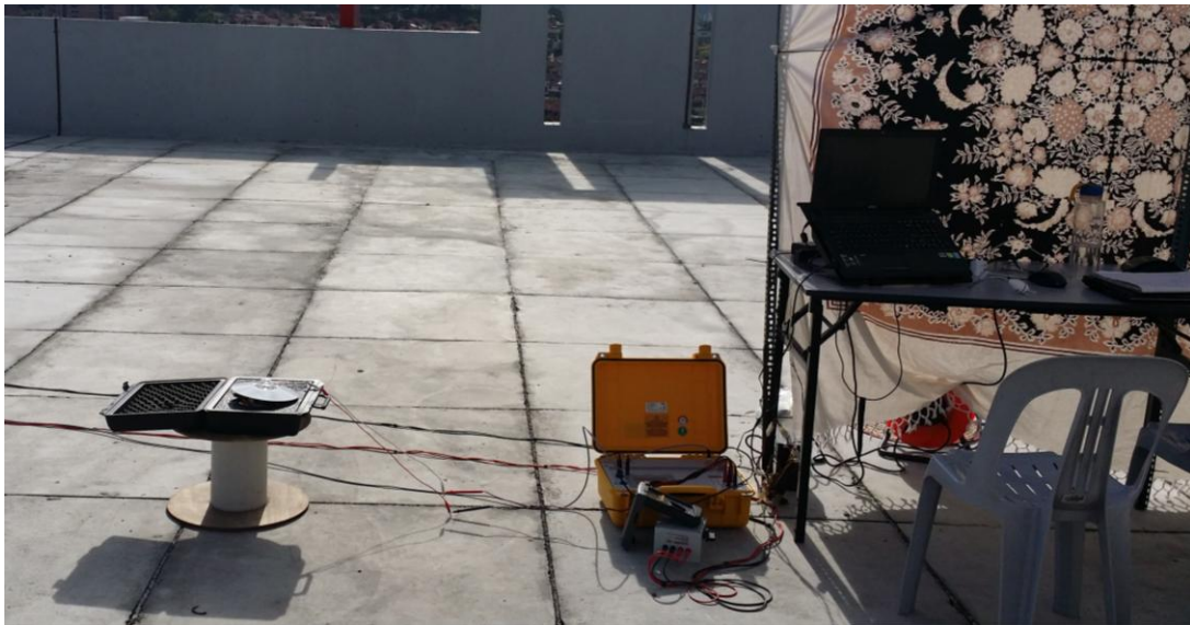
Figure 3.8 : Power and irradiance measurement took by Solar Analyser PVPM 1040
