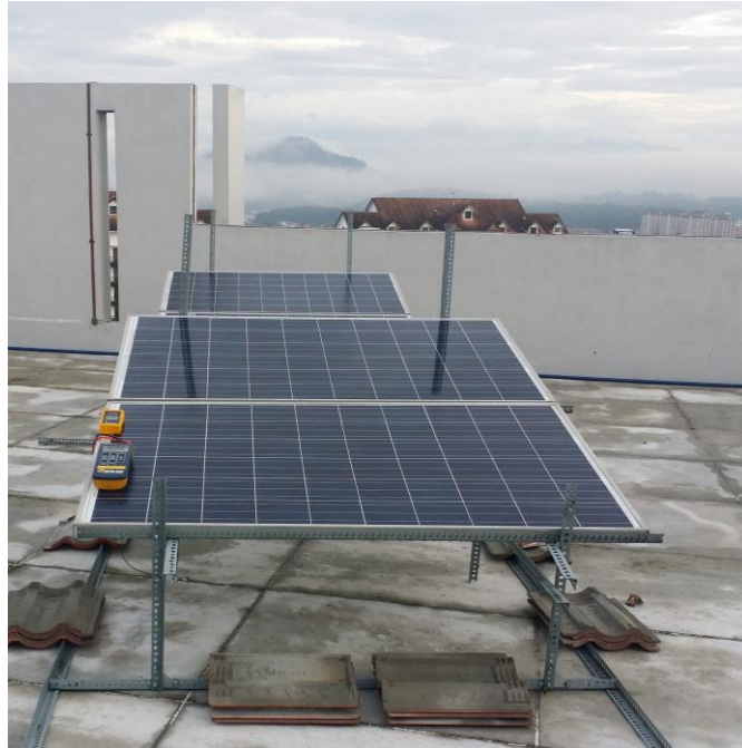
Figure 3.6 : Solar Panel and Structure.
