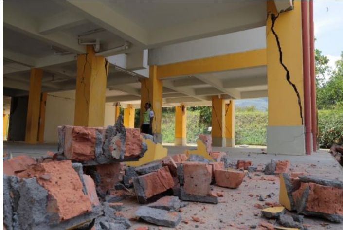
Figure 2.10: Typical Damage of Buildings
