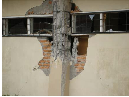
Figure 2.5: Shear Damage due to Short Column Effect in Indonesia (Photo credits: Tim Hart, Lawrence Berkeley National Laboratory)
