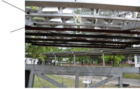
**Figure 4.24: Arrows show the main frame square aluminium bar for supporting the mirror tilting system.**
