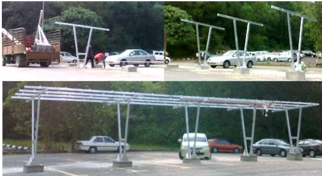
Figure 4.2: Installation of PV Structure
