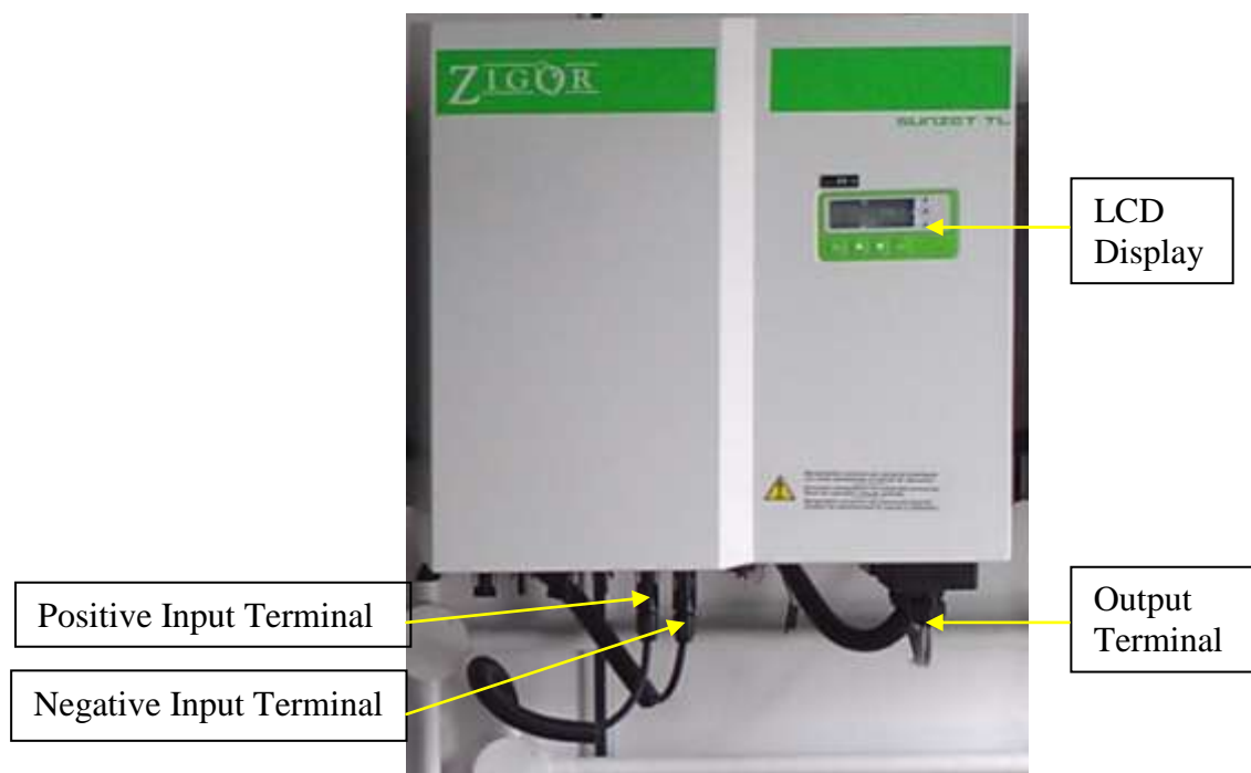
Figure 4.7: PV Inverter
