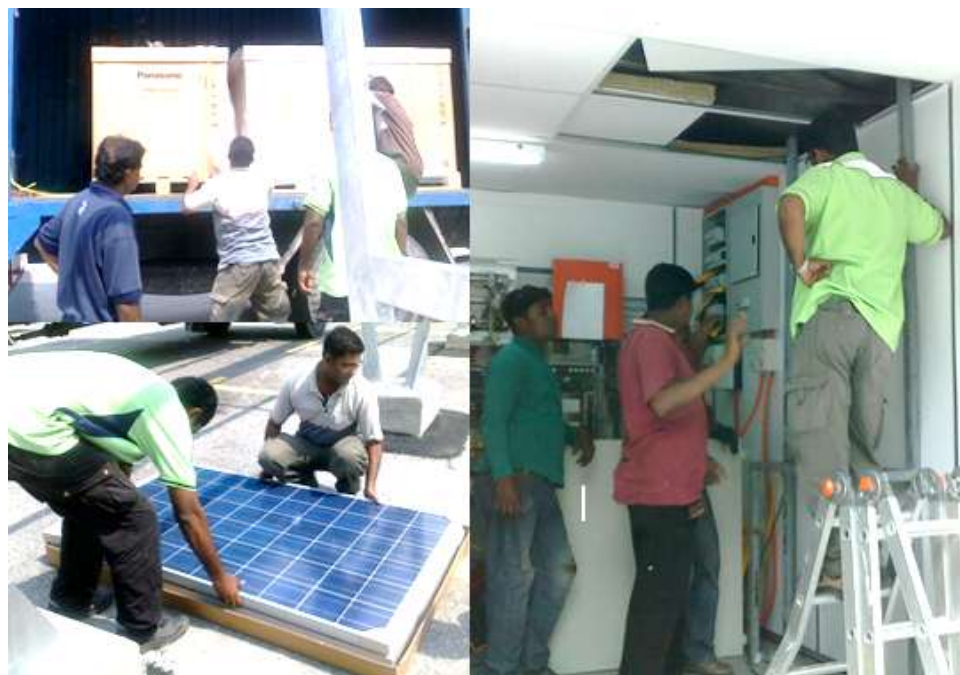
Figure 4.3: Installation of PV System
