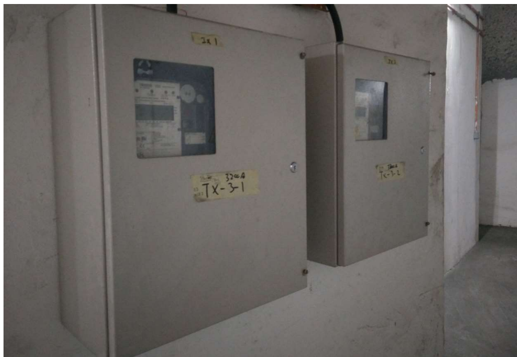
Figure 2.25 Metering panel for TX 3-1 & TX 3-2
