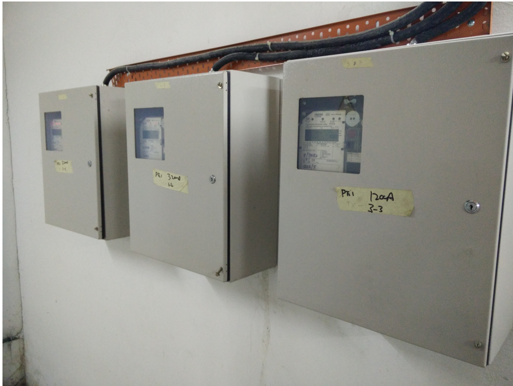
Figure 2.22 Metering panels for TX 1-1, 1-2 & 1.3.
