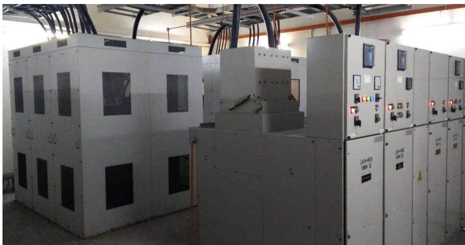
Figure 2.13 Switchgear panels for Substation No.2 and TX2-1 & TX 2-2.
