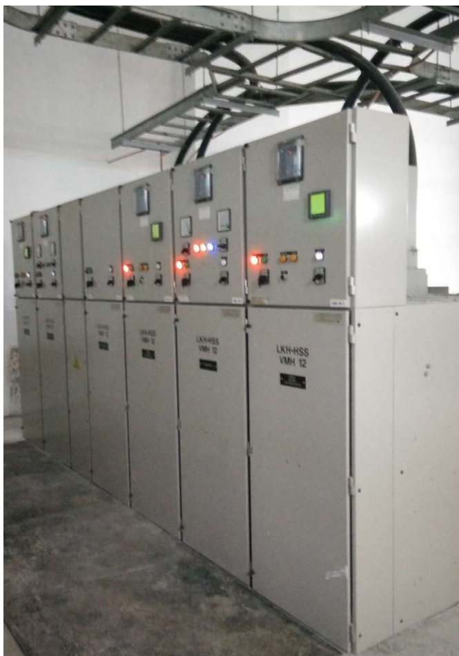
Figure 2.10 Switchgear panels for Substation No.1
