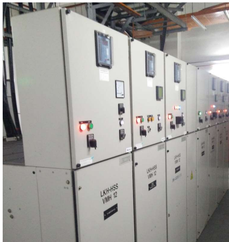
Figure 2.7 Switchgear panels for Substation No.5
