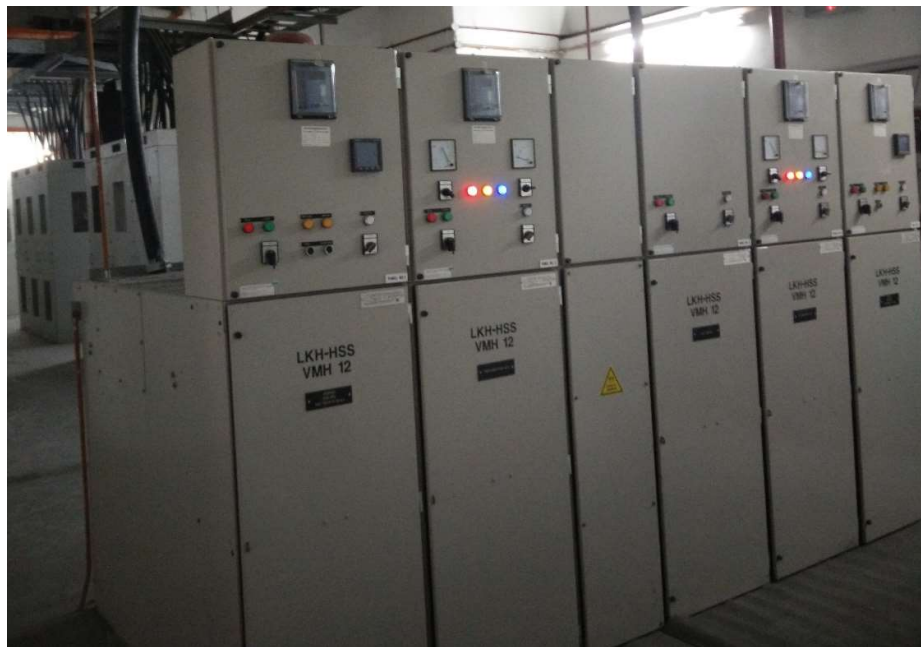
Figure 2.20 Substation No.6 Switchgear panel.
