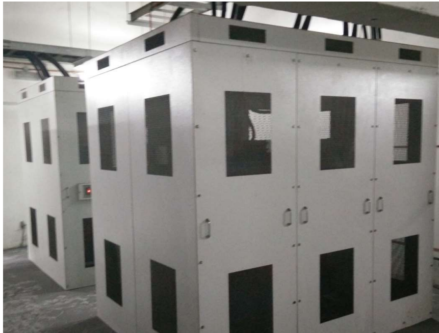
Figure 2.8 Transformers TX 5-1 & TX 5-2.
