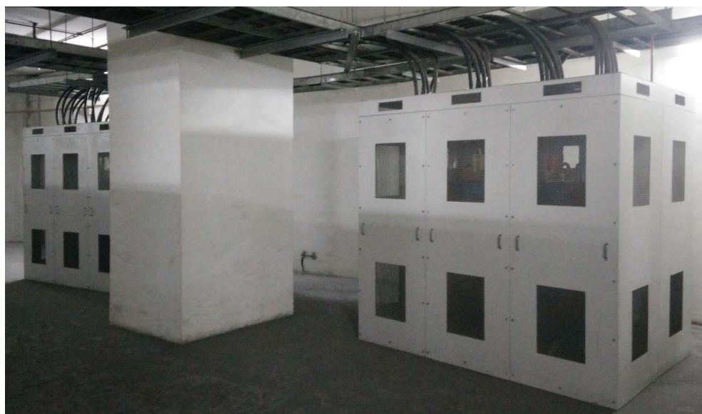
Figure 2.16 Transformer TX3-1 & TX 3-2.
