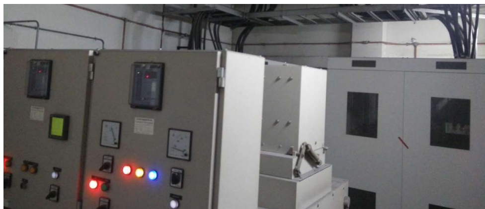
Figure 2.18 Substation No.4 Switchgear panel & Transformer TX1-1 & 1-2
