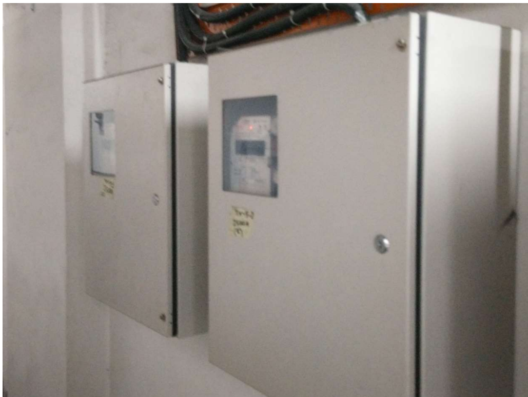
Figure 2.27 Metering panel for TX 5-1 & TX 5-2
