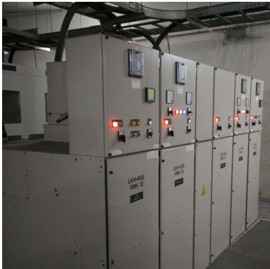
Figure 2.15 Switchgear panels for Substation No.3.
