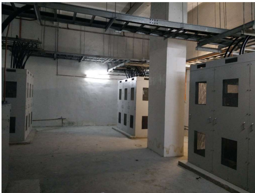
Figure 2.11 Transformers TX 1-1, TX 1-2 & TX 1-3.
