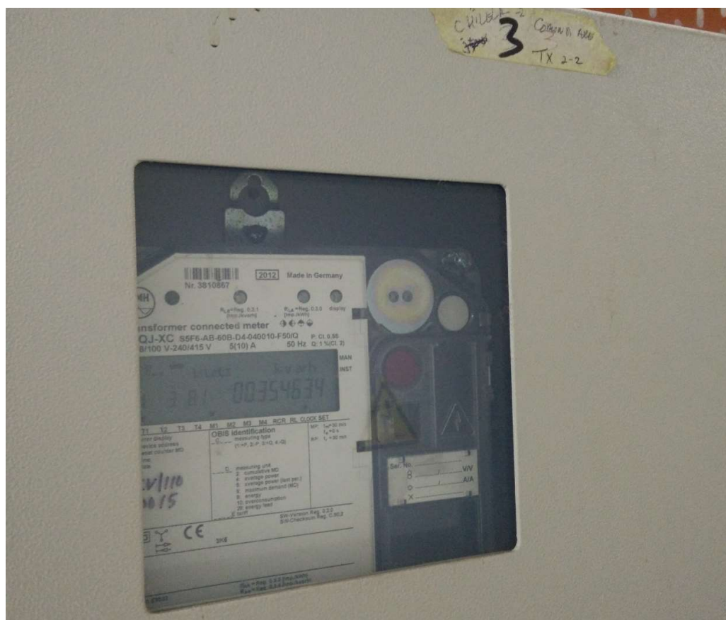
Figure 2.24 Metring panel for TX 2-2
