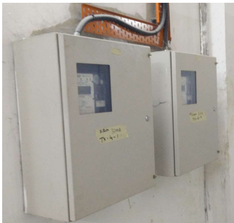
Figure 2.26 Metering panel for TX 4-1 & TX 4-2
