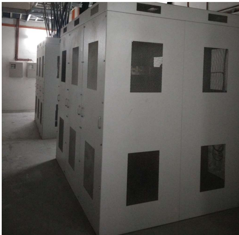
Figure 2.21 Transformer TX 6-1 & 6-2
