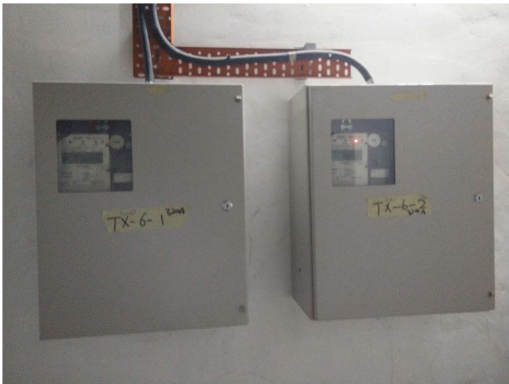
Figure 2.28 Metering panel for TX6-1 & TX 6-2
