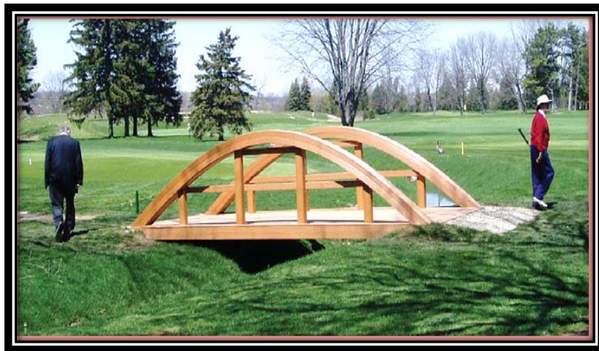
Figure 2.9: Wood Plastic Composite Bridge for Used by Pedestrians and Golf Carts (Pritchard, 2007)
