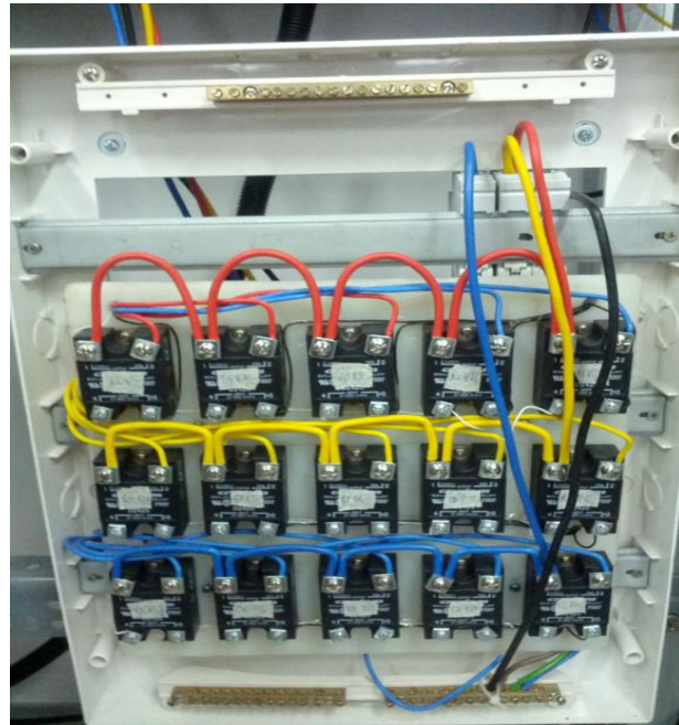
Figure 3.13: Configuration of the SSRs
