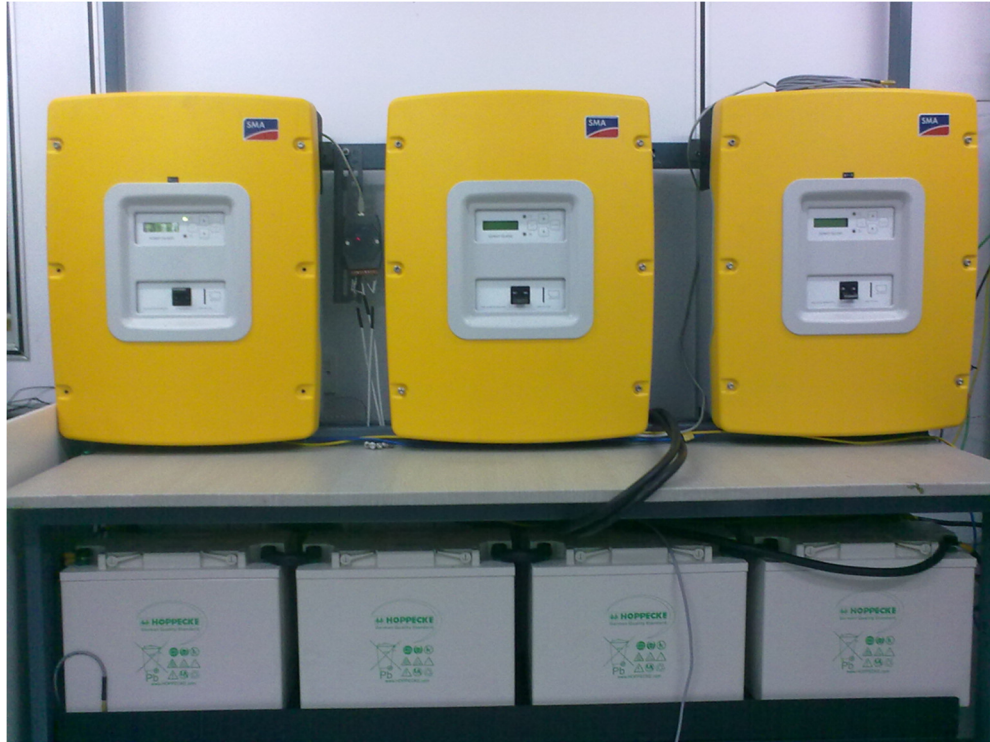
Figure 3.18: Physical 3-phase ESS setup
