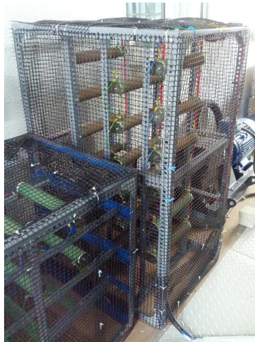
Figure 3.12: Load bank encased in the net
