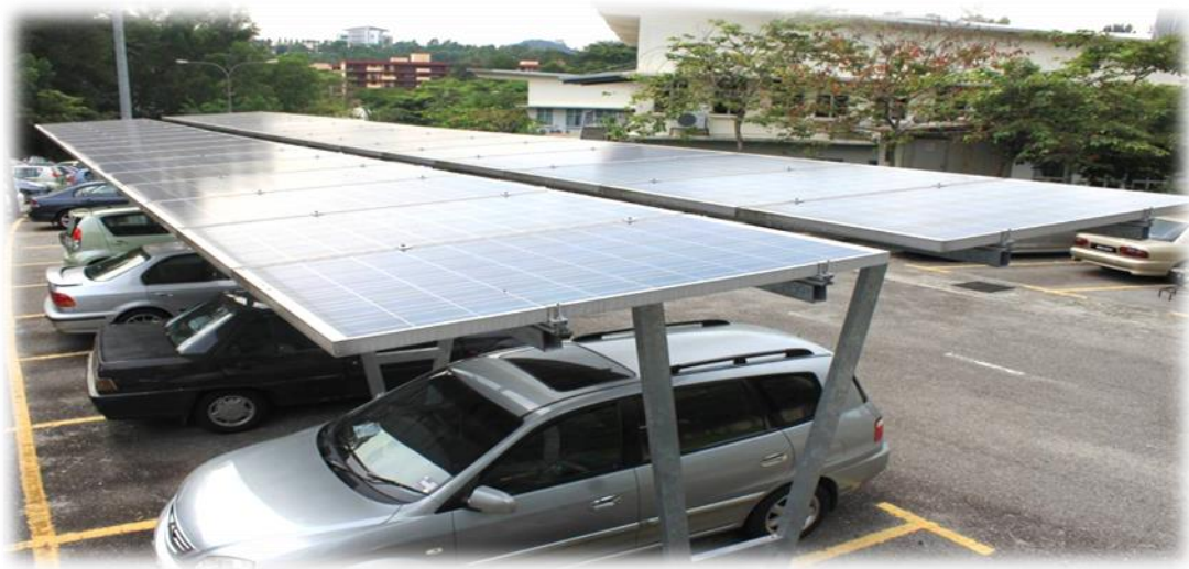
Figure 3.8: Photovoltaic panel mounted on a metal structure
