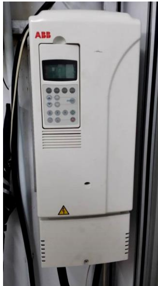
Figure 3.5: Variable speed drive used to drive the induction motor
