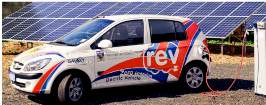
Figure 2: Charging station at EMC Solar, West-Perth
