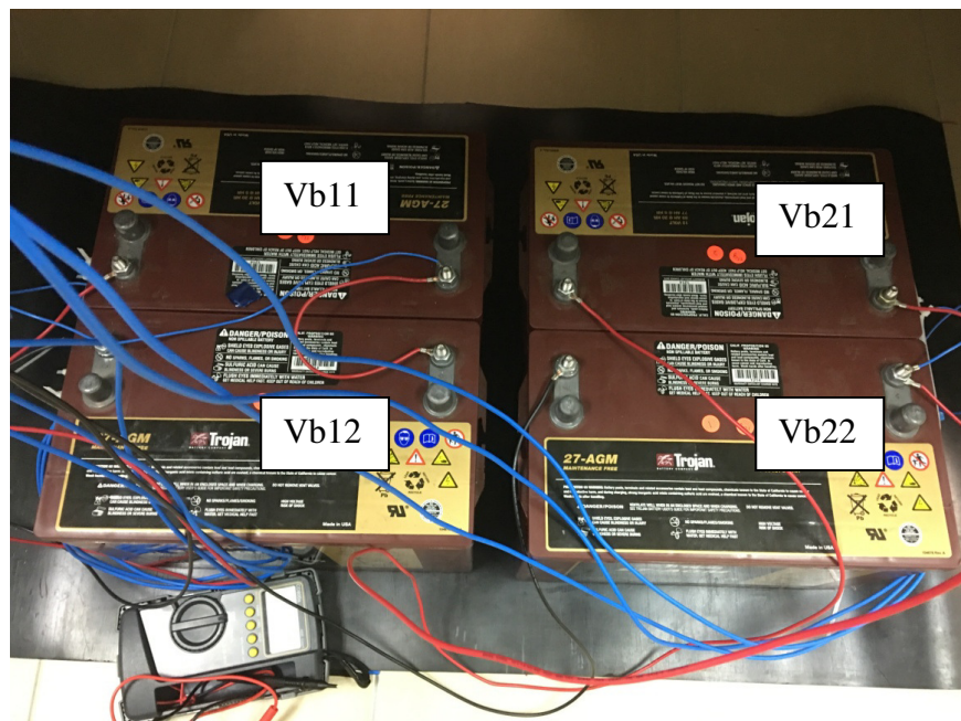
Figure 4.23: Measurement points on batteries
