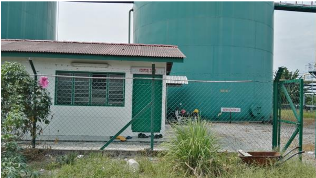
Figure 3.6: Sedimentation Tank No.4 at Tian Siang (Air Kuning) Sdn Bhd
