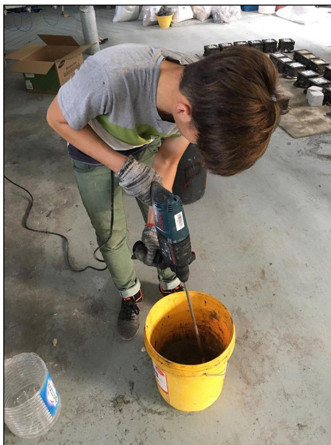
Figure 3.9 Preparation of RePOFA mortar
