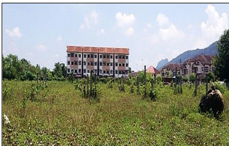
Figure 2.1 Abandoned Housing Project at Eastlake, Kampar in Malaysia
