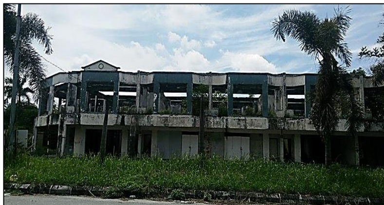
Figure 2.4 Abandoned Shop lots Project at Simpang Pulai, Perak in Malaysia
