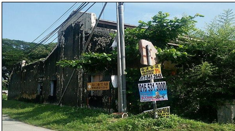
Figure 2.5 Abandoned Housing Project at Ipoh, Perak in Malaysia (All Photos come from own resources)
