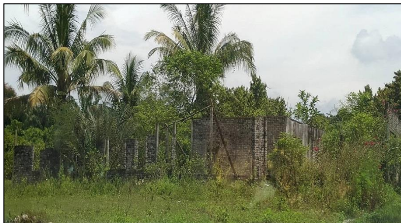
Figure 2.3 Abandoned Housing Project at Kampar, Perak in Malaysia
