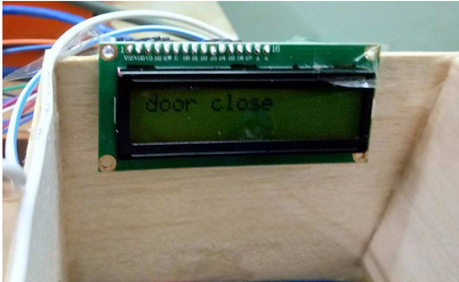
Figure 4.2.37 Status of Door Close on LCD Display
