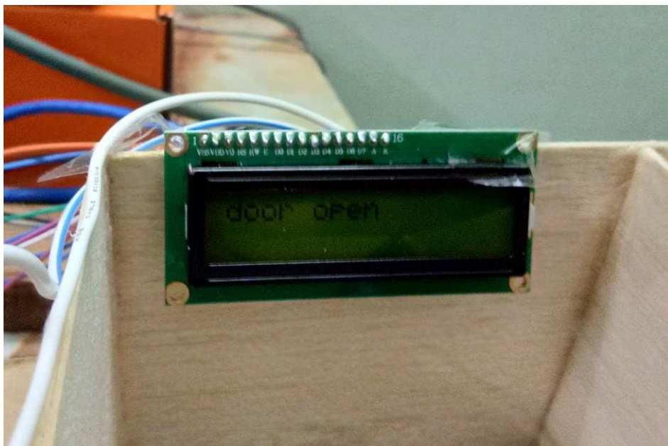
Figure 4.2.34 Status of Door Open on LCD Display
