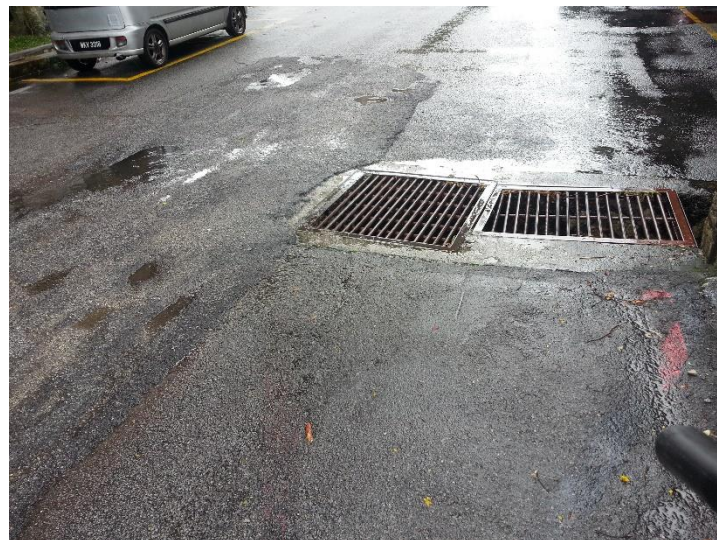
Figure 4-14 Short distance of rough road at top position
