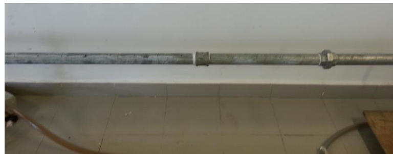
Figure 3.3: Constructed Test Rig
