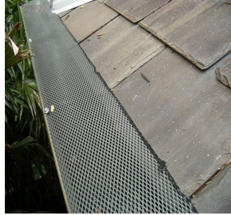
Figure 2.12: Modified roof gutter (Brookes, 2013)
