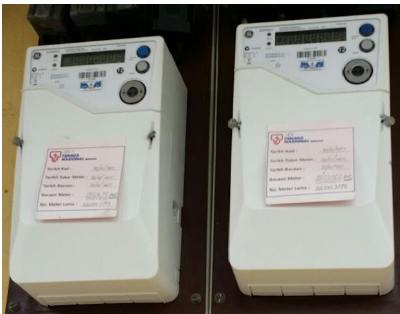
SGM 3031 smart meter made by General Electric.
