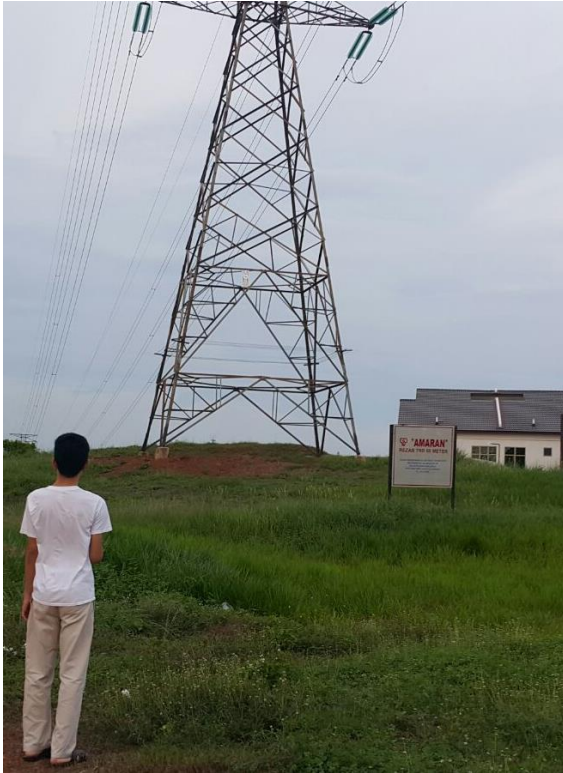
Melaka's 132 kV overhead line
