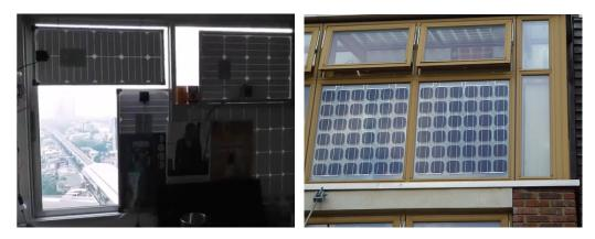
Figure 1.1 C-Si on Vertical Window
