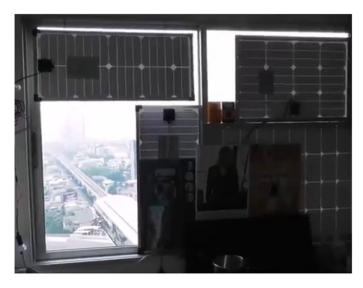
Figure 2.13 Limits the Daylight and Aesthetically Unpleasant
