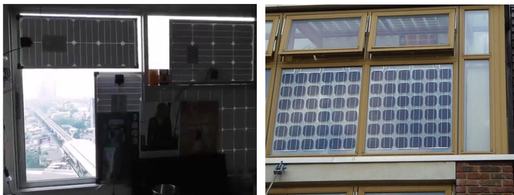
**Figure 1.1 C-Si on Vertical Window**
