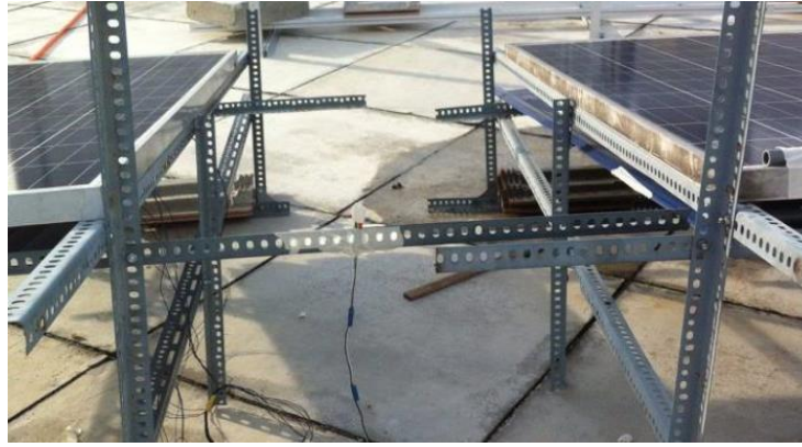
Figure 3.10: DHT22 Position between Both Solar Panels
