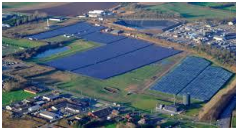
Figure 2.3 Penoles' La Parrena Solar Heating Plant (Golubova, 2016)
