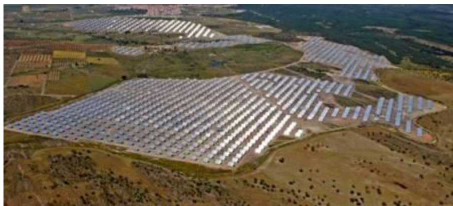
Figure 2.5 Moura photovoltaic power station, Portugal
