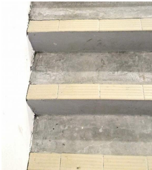
Figure 5.11: Slippery-proof Staircase Finishes in Staircase of UTAR KB Block.
