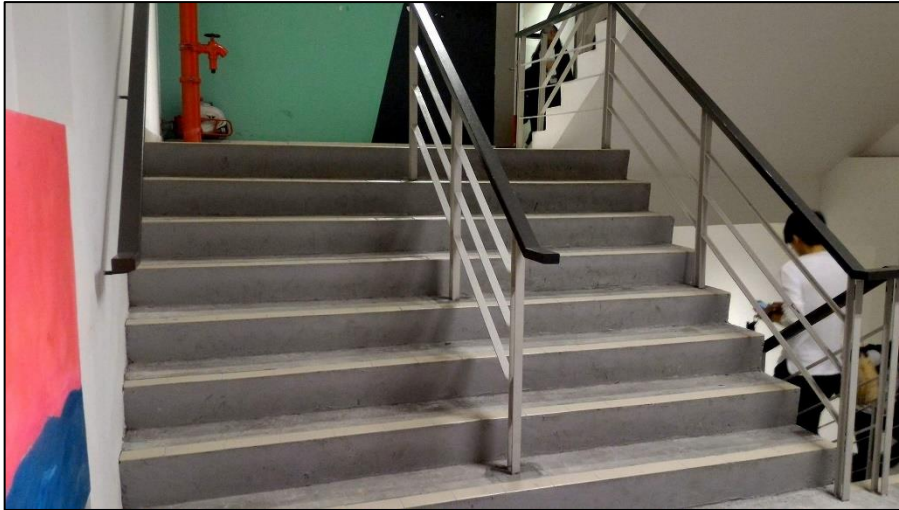
Figure 5.10: Handrails Provided at Staircase in UTAR KB Block.
