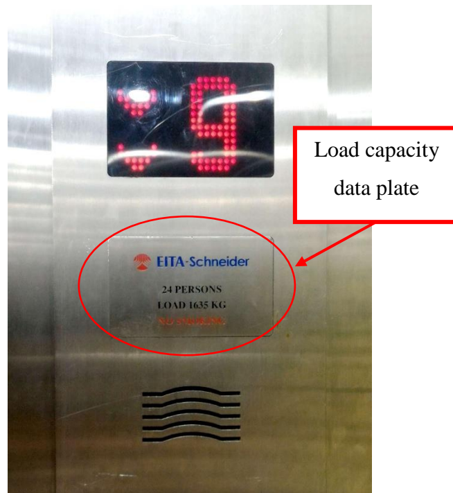
Figure 5.8: Load Capacity Data Plate in a Lift.
