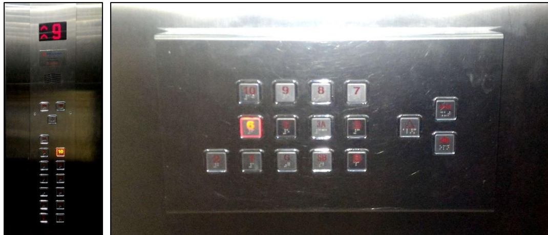
Figure 5.4: Provision of Two Sets of Landing Hall Buttons in the Lift in UTAR KB Block.
