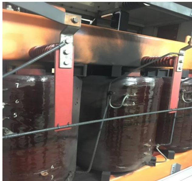
Figure 2.1: Transformer Flashover Due to Inappropriate Protection Scheme
