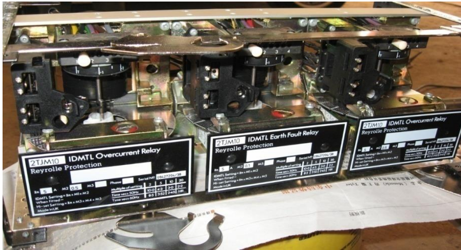
Figure 2.7: IDMT Overcurrent and Earth Fault Relay (Electromechanical)
