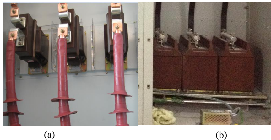
Figure 2.12: (a) Wound Primary Current Transformer (b) Potential Transformer
