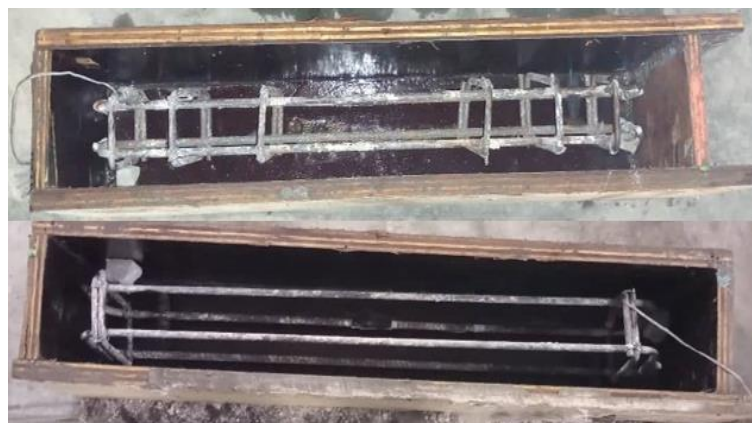
Figure 3.22: Placement of Steel Reinforcement Cage in Beam Formwork
