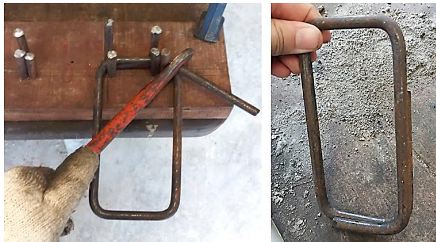
Figure 3.16: Manual Bending of 90° Anchored Shear Link at Bending Platform
