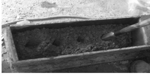
Figure 3.23: Using of Vibrator to Consolidate Fibre Reinforced Concrete Mix
