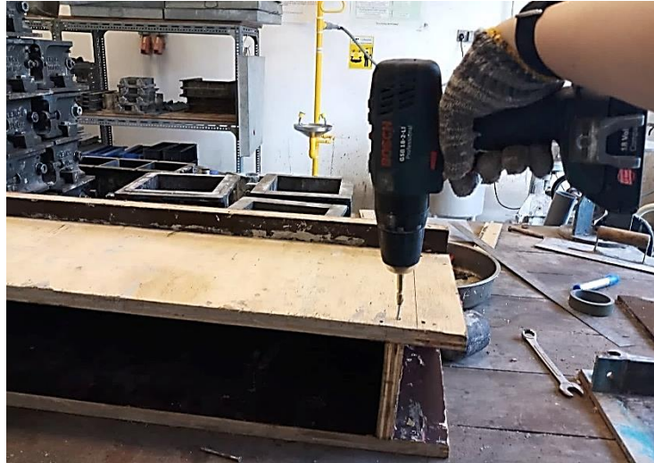
Figure 3.13: Formwork Making According to Dimension of Beam
