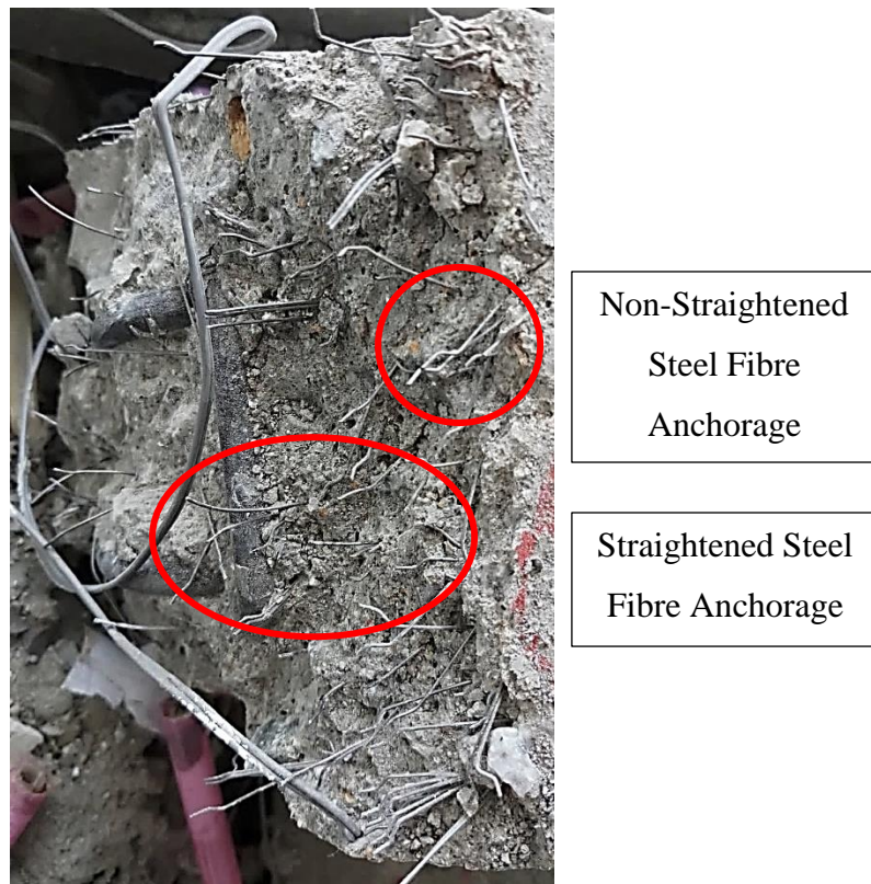
Figure 5.27: Steel Fibre Behaviour on Localized Crack Surface
