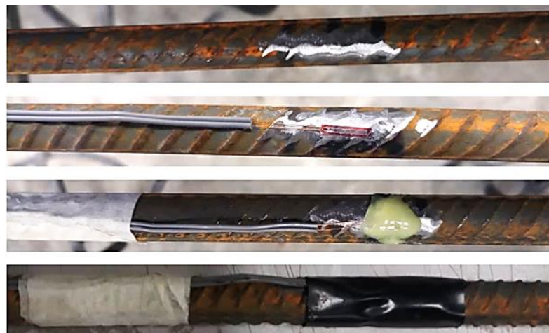
Figure 3.20: Instrumentation of Steel Strain Gauge
