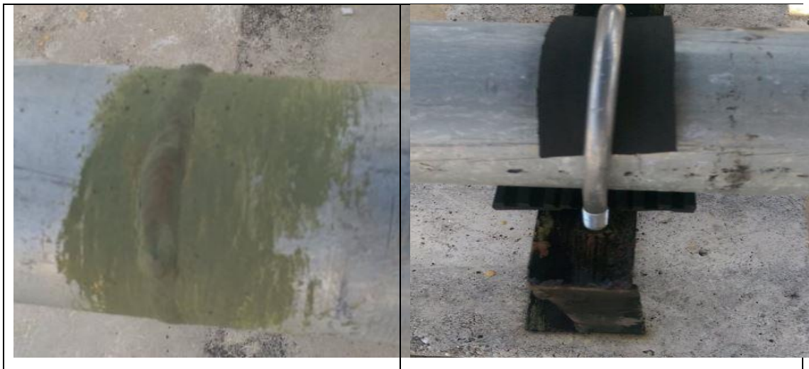
Figure 4-21: Welded spot and Pipeline Holder
