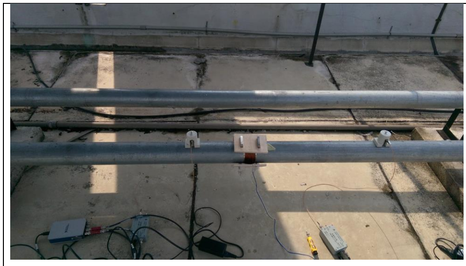
Figure 4-2: Experimental Setup at Rooftop
