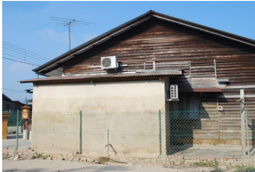
Figure 2.25: Scene after flood in Gemas Bahru
