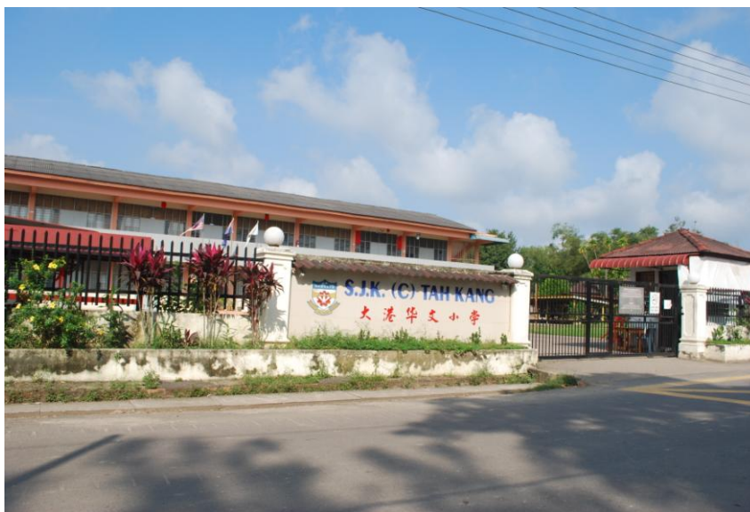
Figure 2.16: Tah Kong primary school in Gemas Bahru
