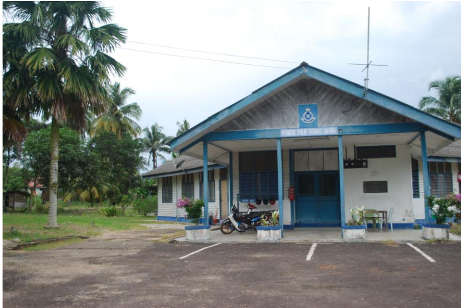
Figure 2.21: Police station in Gemas Bahru
