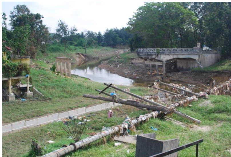
Figure 2.10: The historial destroyed bridge
