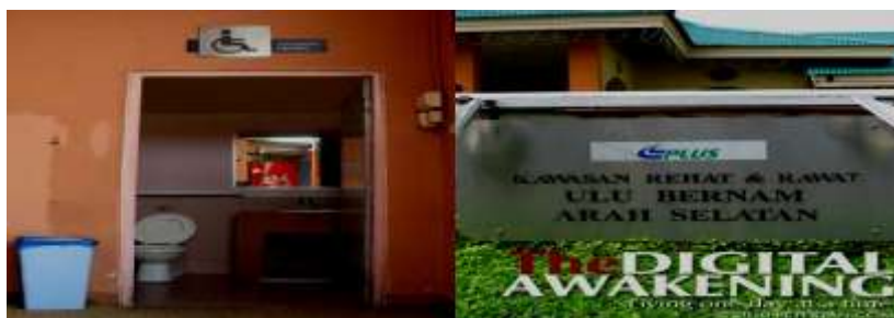
Figure 1 Toilet for disabled at Ulu Bernam RSA Southbound (Source: Peter Gabriel Tan, 2010)
