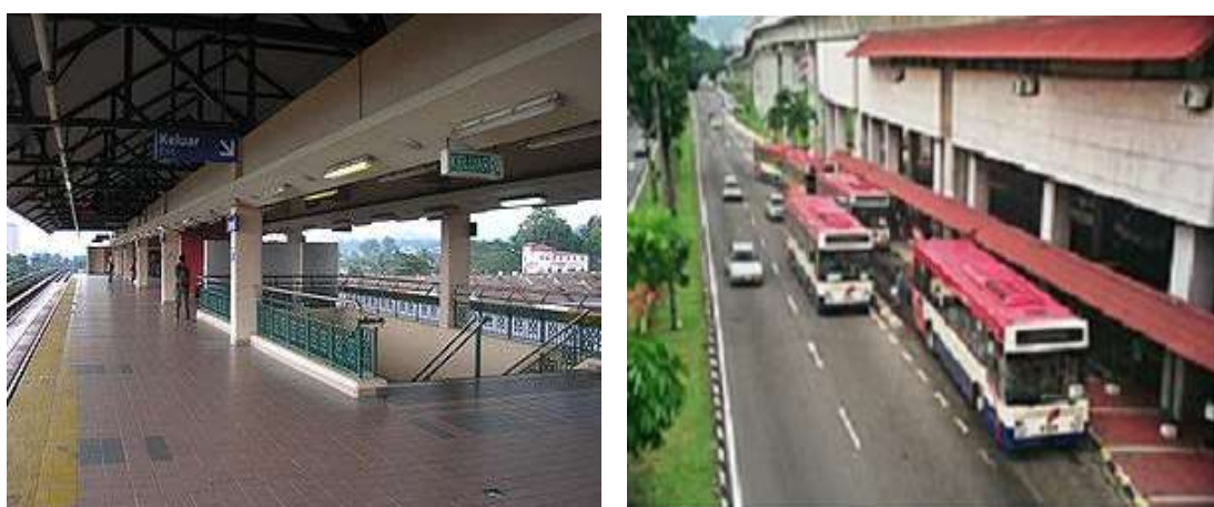
Figure 48 Wangsa Maju LRT station
