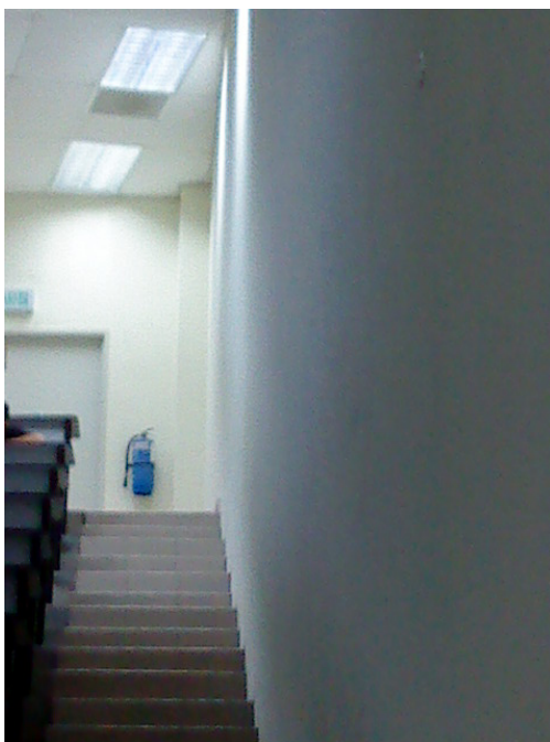
Figure3-2: Lecture hall's wall
