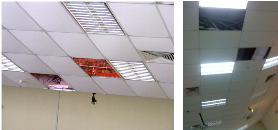
Figure 4-10: Opened hole at lecture hall
