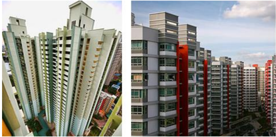
Figure 4.40: Current HDB housing are well planned and colorful. Image from : < https://www.teoalida.com/world/ >
