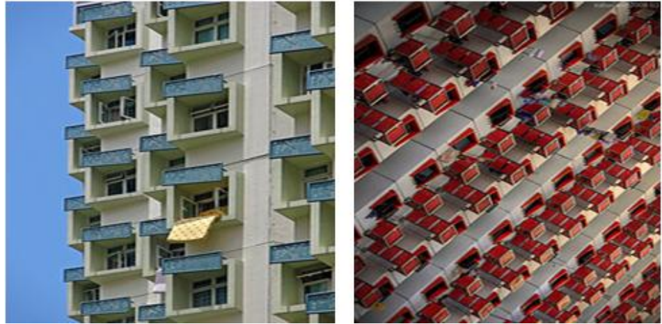
Figure 4.42: Additional screen laundry design in current HDB housing. Image from : < https://www.teoalida.com/world/ >
