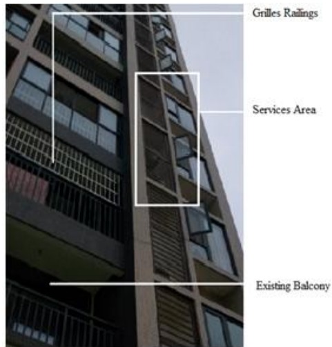
Figure 6.2: Semi enclosed screening grilles at exposed balcony. Image from own source.
