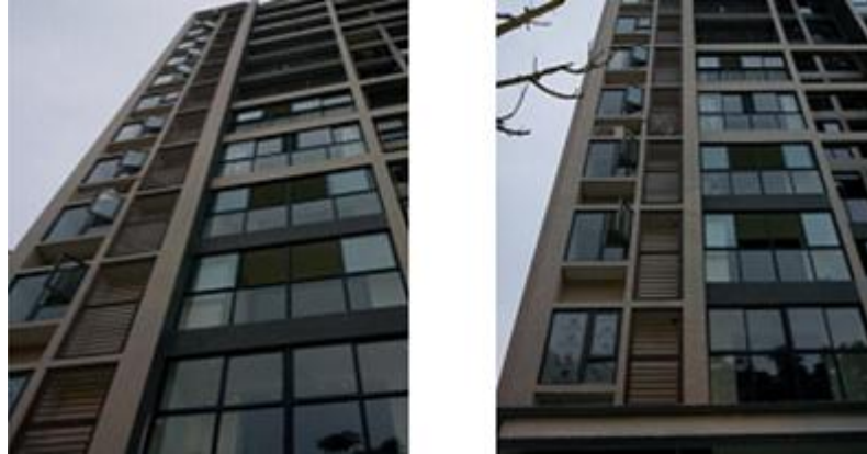
Figure 6.4: Glazed installations at the exposed balcony add character to the building. Image from own source.
