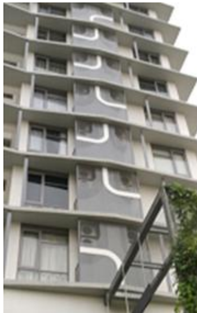
Figure 6.7: Screen panels at service area add character while concealing the laundry. Image from own source.
