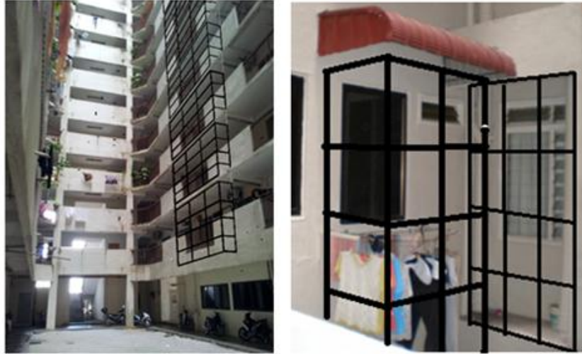
Figure 2.14: Proposed RACD inside the Cage Grilled where laundry can dried faster. Image own source.
