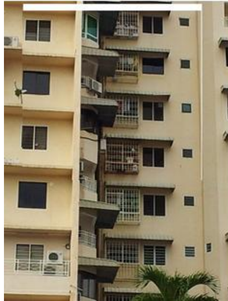
Figure 6.14: Proper design, control and standardization of caged laundry appear to be more orderly. Image from own source.
