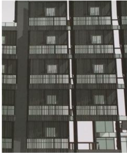
Figure 6.20: Standardized grilles cage compliments the overall building envelope. Image from own source.
