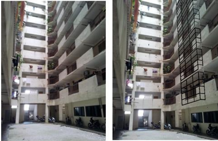
Figure 6.16: Proposed vertical cage grilles or perforated prefab panels grilles. Image own source.
