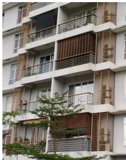
Figure 4.19: Exposed balcony is a common laundry location. Image from own source.
