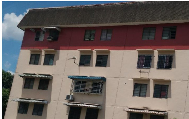
Figure 6.11: Cage laundry installed at window openings. Image from own source.
