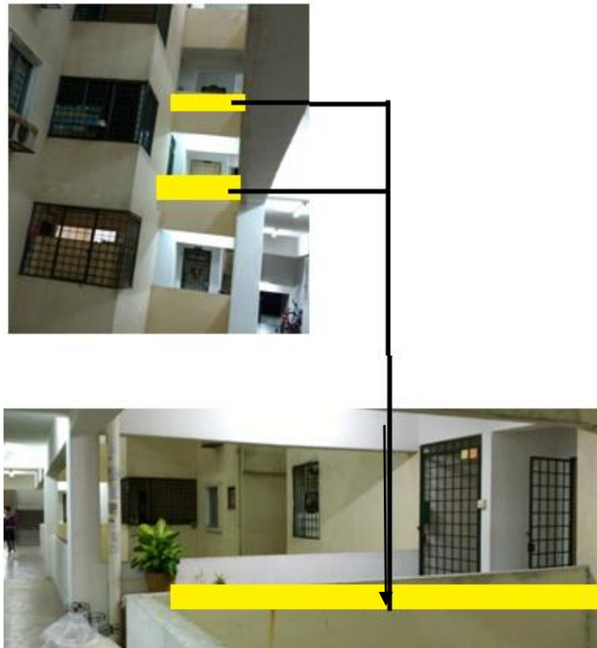
Figure 4.25: Typical Alternate Air Well of Double Sandwich Block (DSB) and laundry locations. Image from own source.
