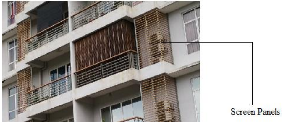
Figure 6.10: Metal screen panels at balconies. Image from own source.
