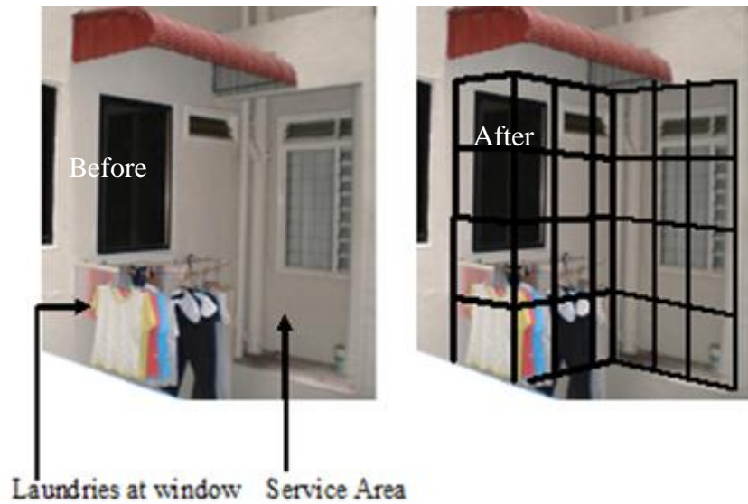
Figure 6.18: Installation of individual cage grilles for the punctuated air-well. Image from own source.
