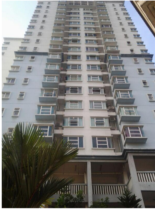
Figure 4.34: Middle class private development, no laundry area provided. Image from own source.
