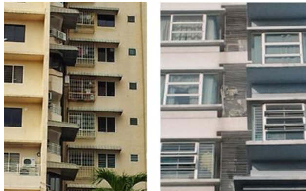
Figure 4.18: Cage laundries and screen panels for laundry location. Image from own source.
