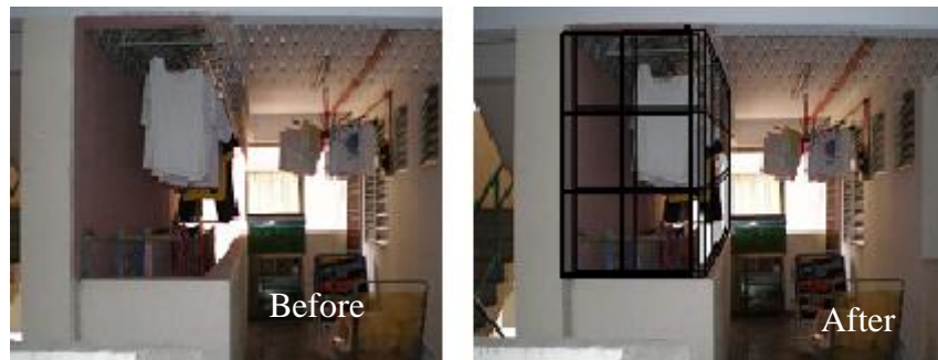
Figure 6.19: 'Before' and 'After' views of cage laundry along the Common corridor for the corner unit. Image from own source.
