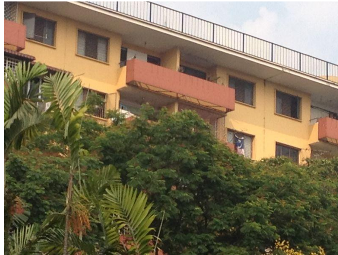
Figure 4.36: Improvised balcony with panels as screening device for unsightly hanging laundries. Image from own source.
