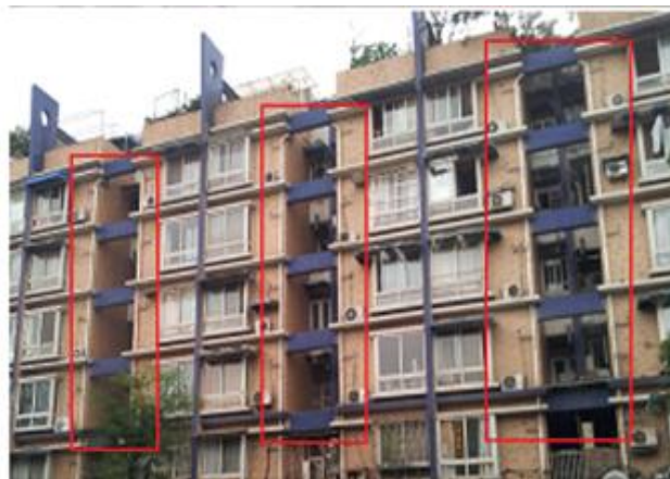
Figure 6.9: Exposed screen panel for air-condensers within window vicinity. Image from own source.
