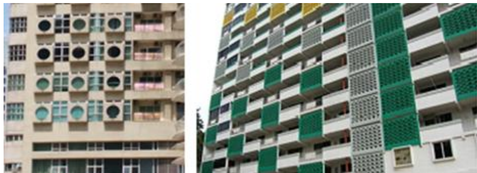
Figure 6.6: Precast screen panels with geometry design enhance the overall building façade. Image from own source.
