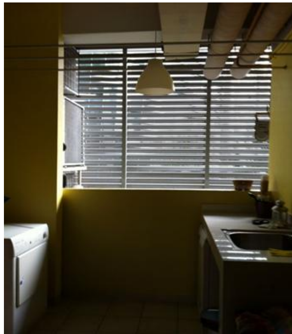
Figure 4.30: Screen panels to screen off laundries area at private housing. Image own source.
