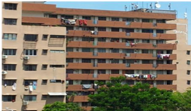
Figure 4.28: A common sight to see laundry exposed along common corridors. Image from own source.
