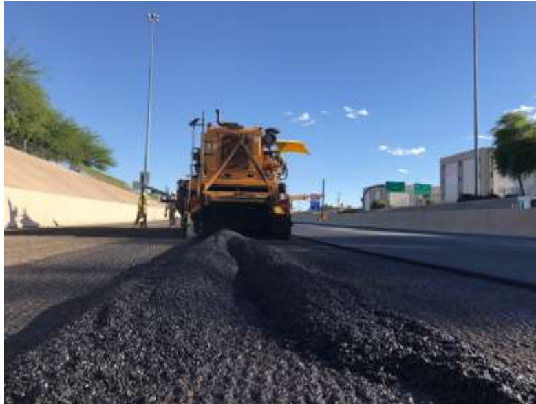
Figure 2.7: Rubberized Asphalt Pavement (ADOT, 2017).
