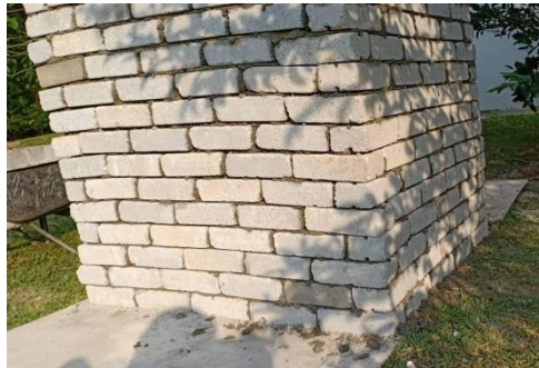
Figure 4.18 : Well-constructed Brick Wall
