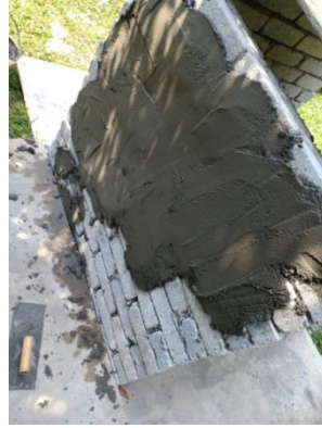
Figure 4.19 : The Process of Plastering
