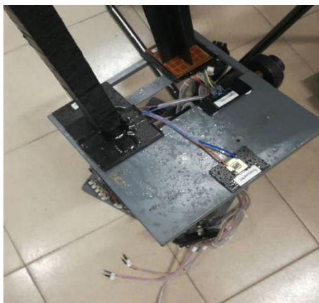
Figure 5.2: The Solar Tracker Was Wet Due To Heavy Rain
