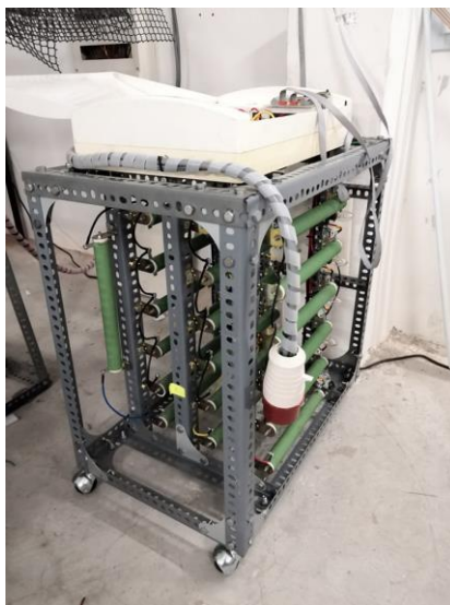
Figure 3.23: 3kW Load Bank Module
