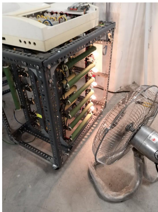
Figure 3.26: Testing resistors connection
