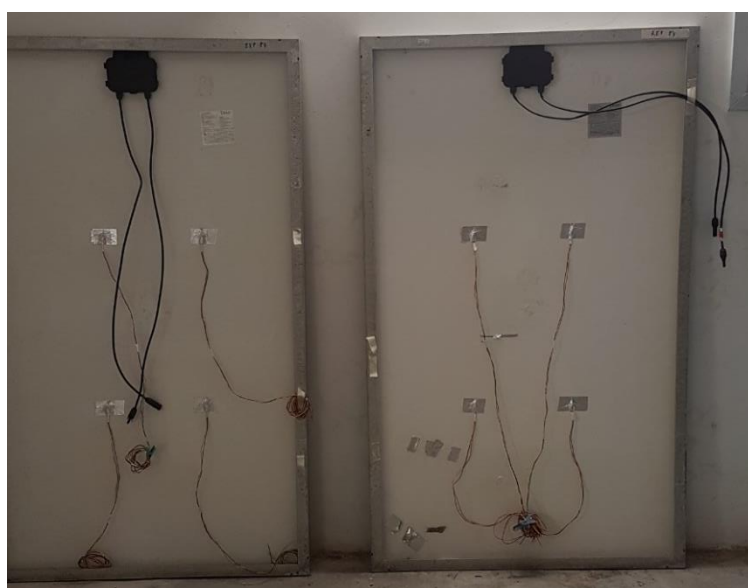
Figure 3.4.1.3: Attachment of DS18B20 Temperature Sensors underneath PV panels.
