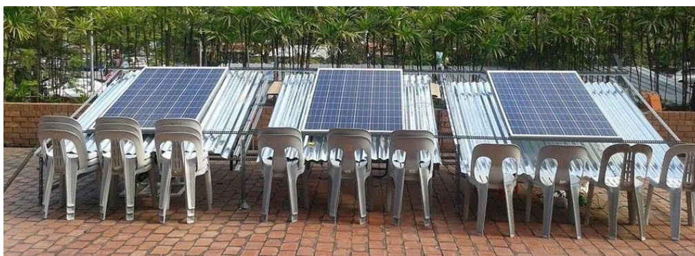
Figure 2.2.4.1: Metal-Deck Roof Mock-Up Experiment in Bandar Sg Long, Selangor. (Chew, 2015)
