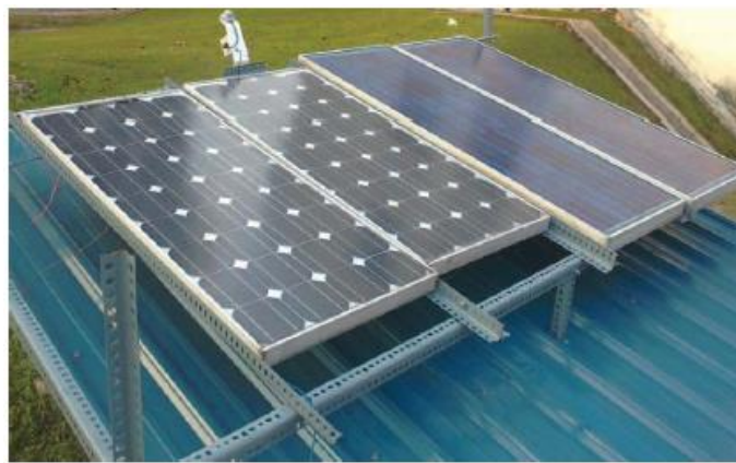
Figure 2.2.2.1: Metal-Deck roof Mock-Up Experiment on campus in Shah Alam, Selangor. (Zakaria et al., 2013)
