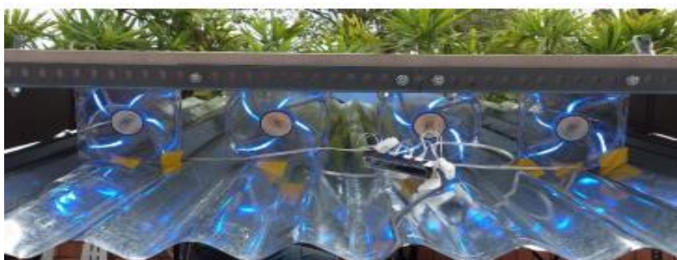
Figure 2.2.5.2: Fan System beneath the BAPV system. (Chong, 2015)
