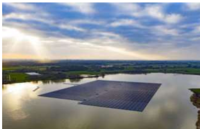
Figure 2.6: Floating solar farm in Netherlands (Mathis, 2020)
