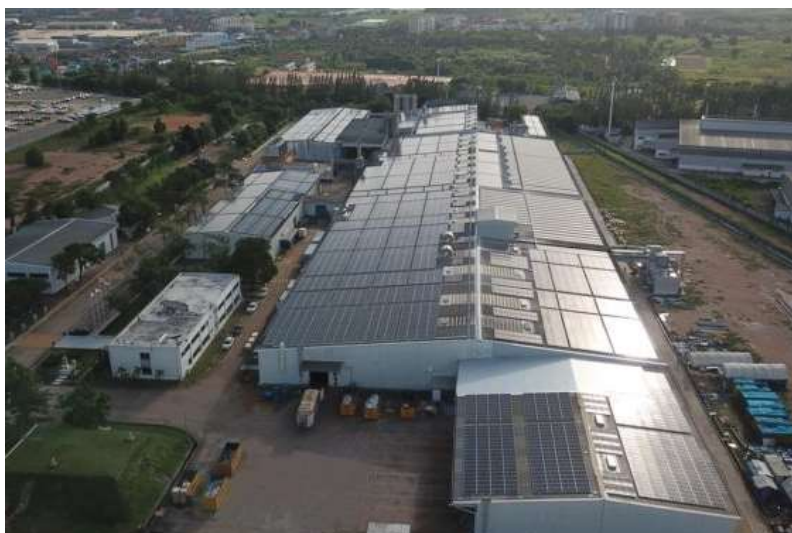
Figure 2.2: Rooftop solar system in Rayong, Thailand (Symbior Solar, n.d.)
