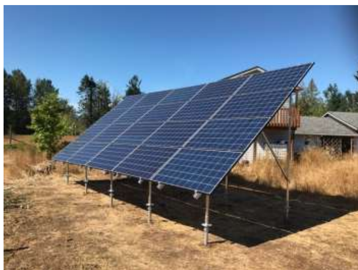
Figure 2.1: 5.5 kW ground-mounted solar system in Canada (Shift Energy Group, n.d.)
