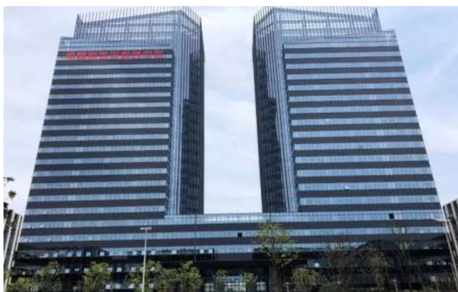
Figure 2.5: BIPV with a total power capacity of 460 kW in Nanchang, China (Djunisic, 2019)
