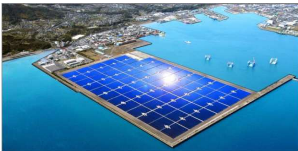
Figure 2.4: Kagoshima Nanatsujima Offshore solar PV plant in Japan (Kumar, Shrivastava and Untawale, 2015)
