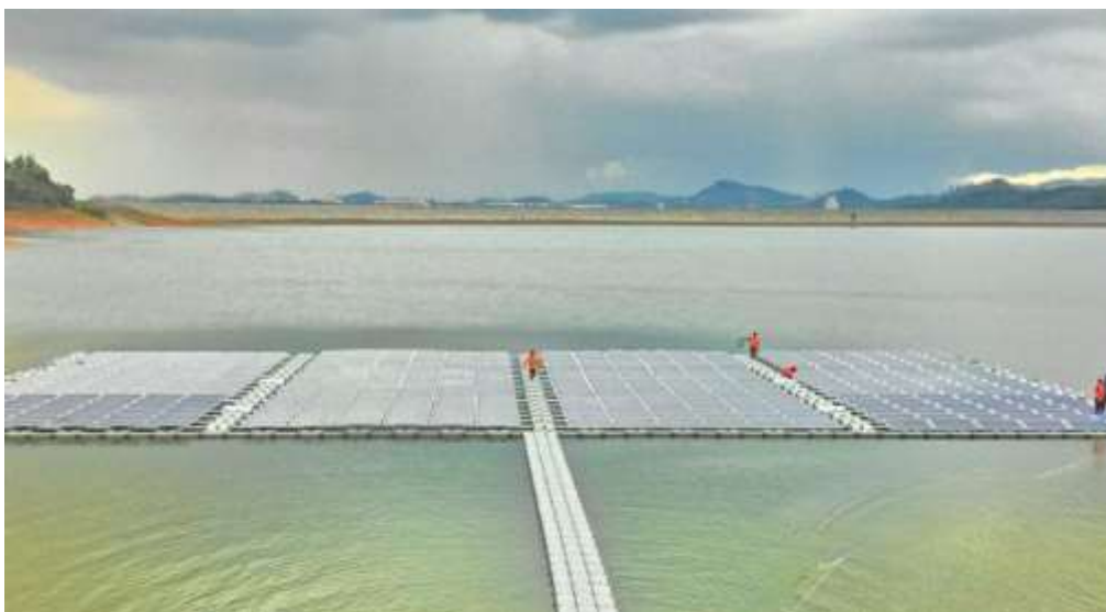
Figure 1.1: Malaysia's first floating solar plant in Sungai Labu (Ciel & Terre, n.d.)
