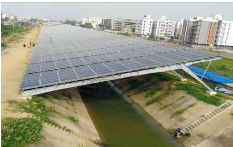
Figure 2.3: Canal top solar plant in Gujerat, India (Srivastava, 2016)
