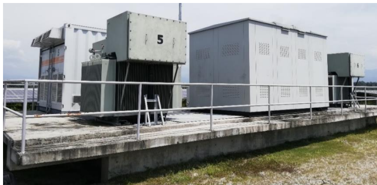
Figure 1.3: Central inverter for LSS that costs millions of ringgit.
