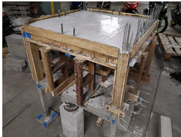
Figure 3.7: Concrete Casting of Second Level Slab and Beam.
