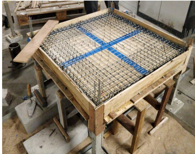
Figure 3.4: Installation of Slab and Beam Reinforcement into Plywood Formwork.
