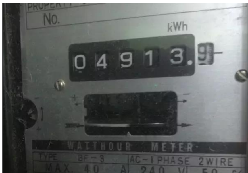
Figure A.13: Utility meter 13.
