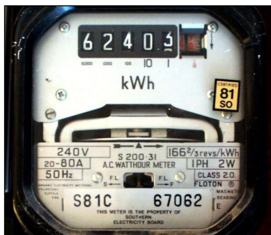
Figure A.20: Utility meter 20.
