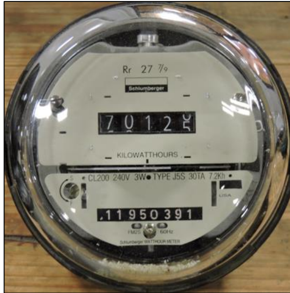
Figure A.18: Utility meter 18.
