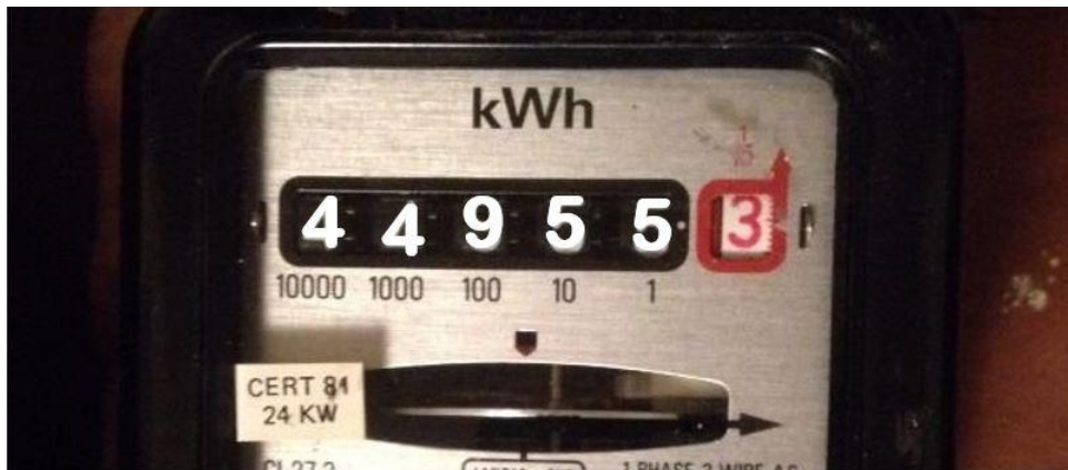
Figure A.10: Utility meter 10.
