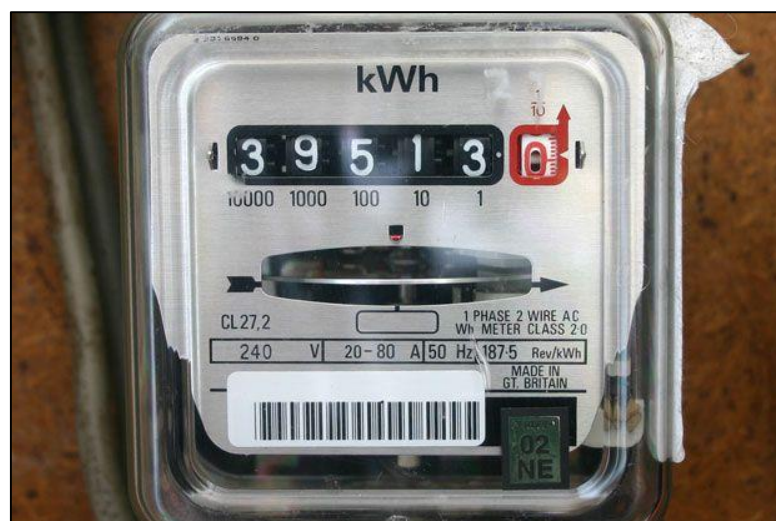
Figure A.17: Utility meter 17.
