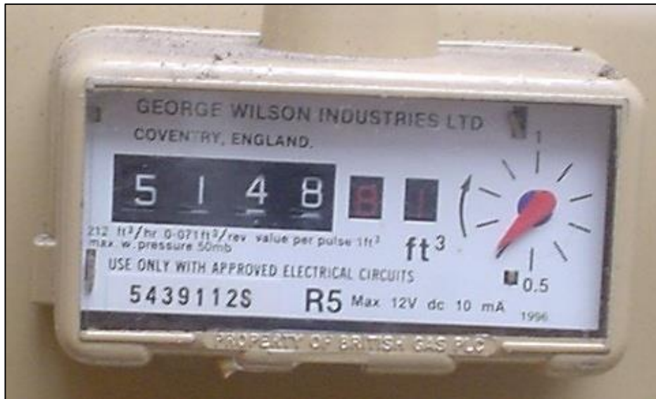
Figure A.7: Utility meter 07.
