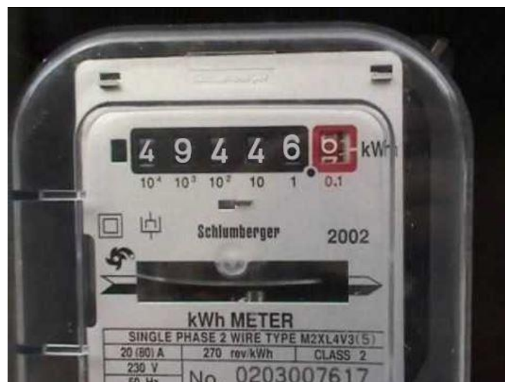
Figure A.14: Utility meter 14.
