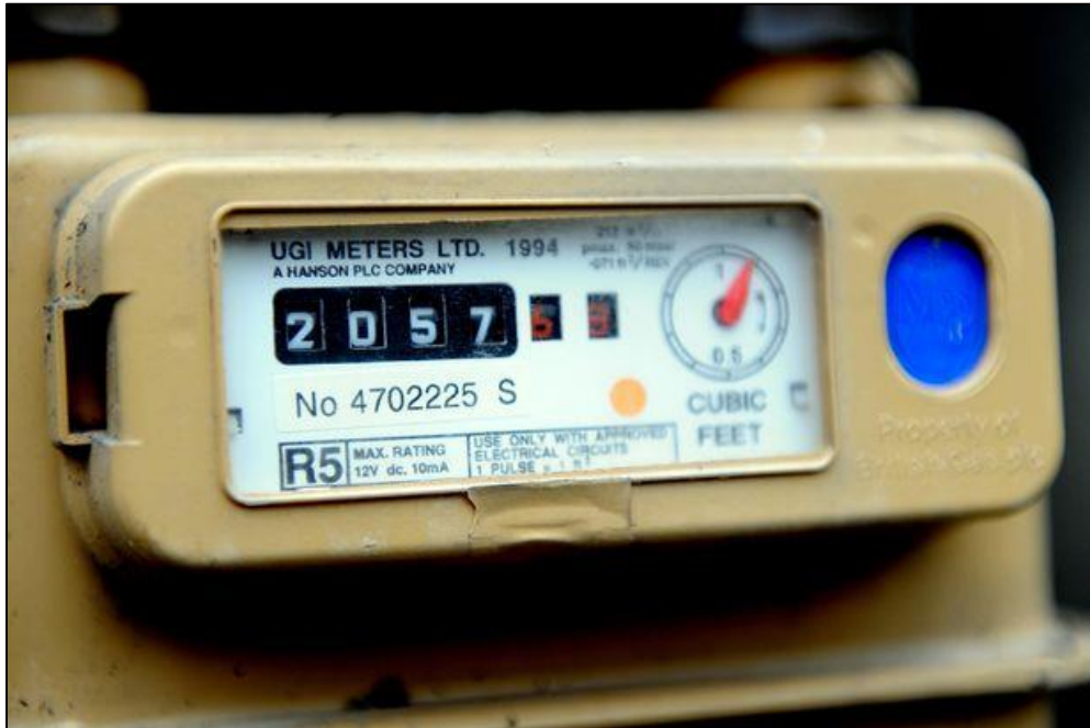
Figure A.5: Utility meter 05.
