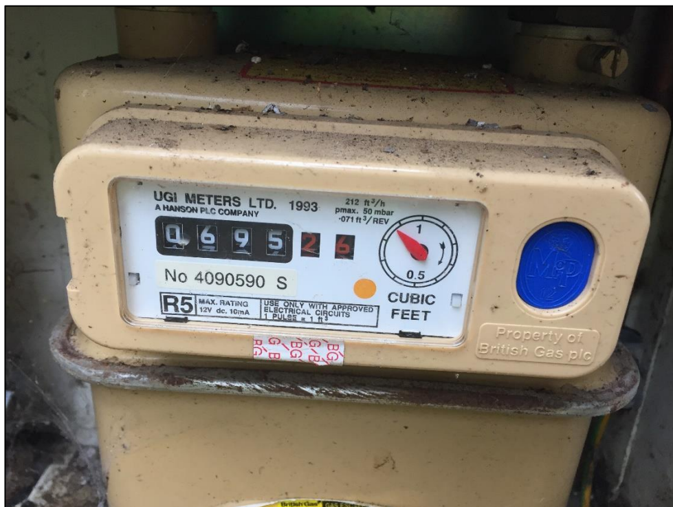
Figure A.6: Utility meter 06.
